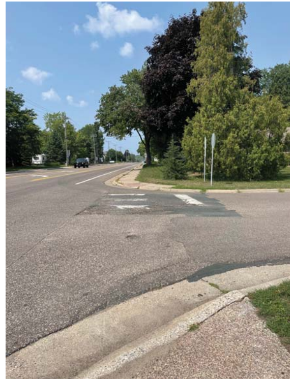
The corridor lacks consistent ADA compliant pedestrian ramps as shown in the example above and to the right at Medicine Lake Rd (CSAH 70) and Hampshire Ave.
