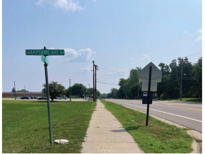
The nearest crossing for the Neill Elementary School is Hampshire Ave N and Florida Ave N. This project will include additional crossing enhancements along the corridor as warranted.
