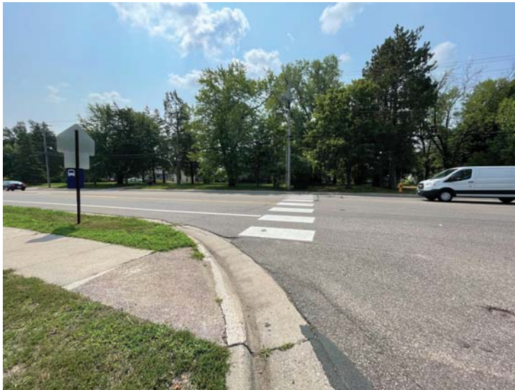
The corridor lacks consistent ADA compliant pedestrian ramps as shown in the example above and to the right at Medicine Lake Rd (CSAH 70) and Hampshire Ave.
