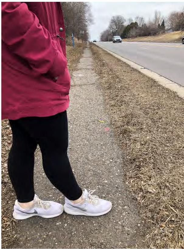
Fig 3 and 4, W 94<sup>th</sup> to W 98<sup>th</sup> Streets, West side – Example of Narrow trail (approx. 2 1/2 ' wide, deteriorated pavement, narrow boulevard
