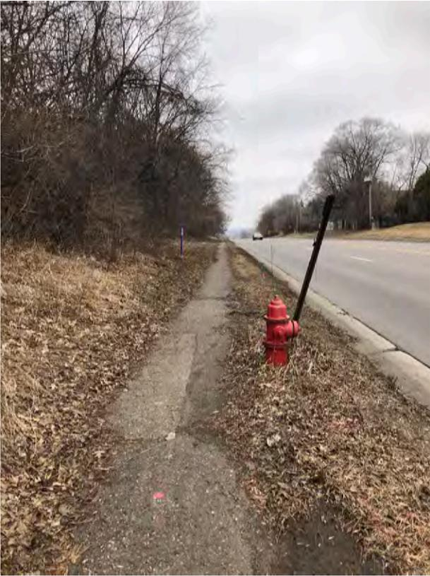
Fig 2. W 94<sup>th</sup> to W 98<sup>th</sup> Street, West side – Examples of narrow path, deteriorated pavement, and clear zone obstructions
