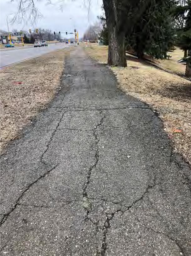
Fig 1. W 94<sup>th</sup> to W 98<sup>th</sup> Street, West side –Examples of deteriorated subgrade and pavement
