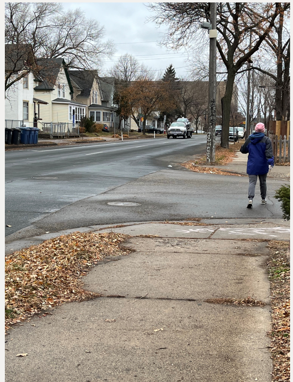
28th Street East at 14th Avenue
