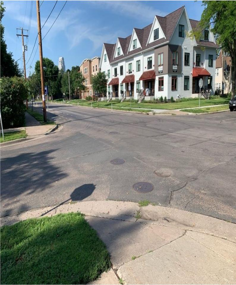
Photo of the intersection of 10th Ave SE and 7th St SE showing ADA non-compliant pedestrian ramps and a wide, difficult to cross street.
