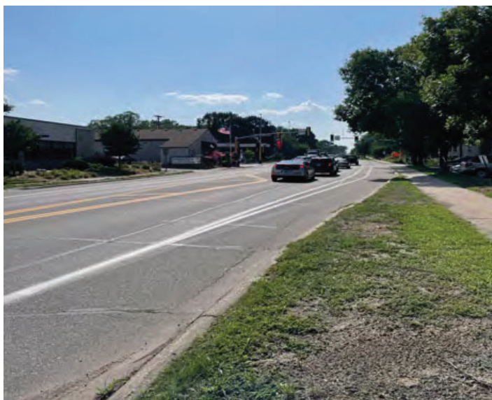
Existing bike infrastructure pictured above east of the Dakota Ave intersection.
