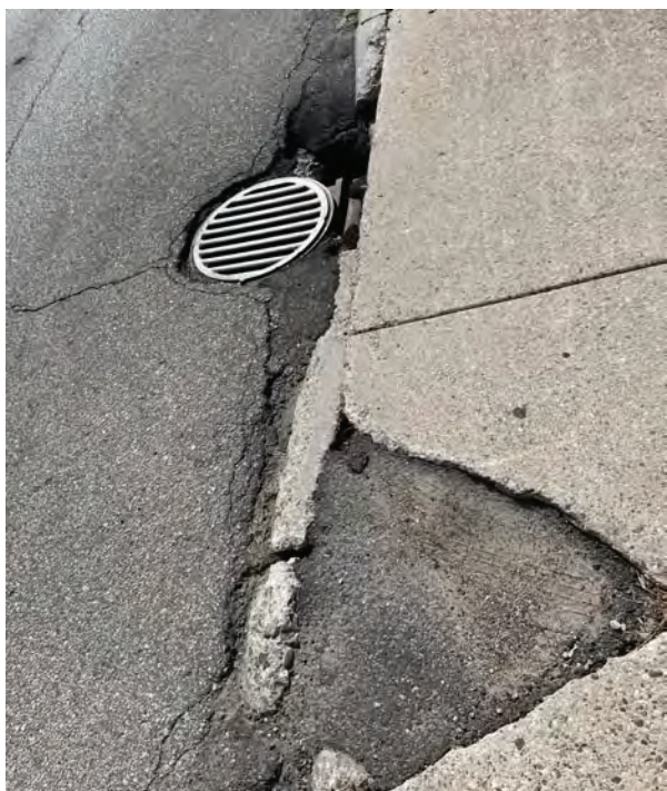
Many sections of the existing roadway, sidewalk and gutter pan are experiencing significant cracking and are in generally poor condition, as demonstrated above.
