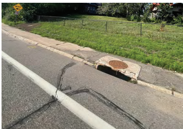
Many sections of the existing roadway, sidewalk and gutter pan are experiencing significant cracking and are in generally poor condition, as demonstrated above.
