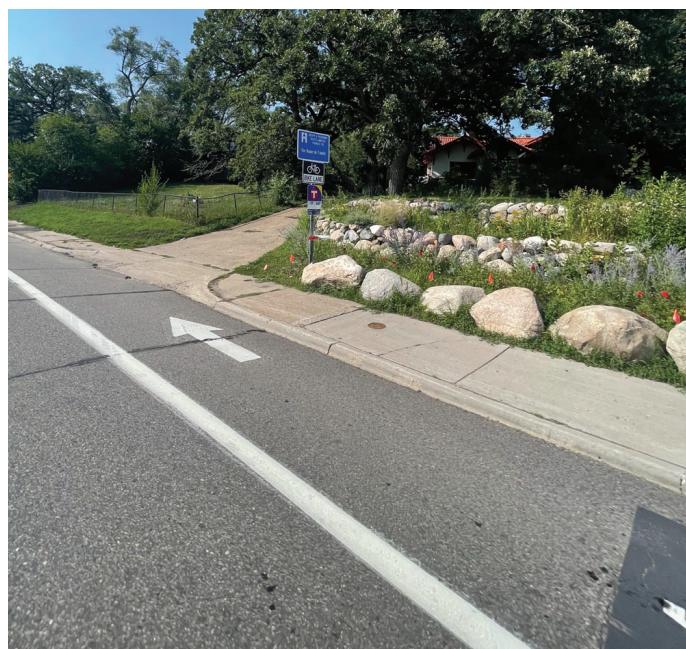
Existing on-street bike infrastructure does not accommodate all ages and abilities, and sidewalks are at back of curb in some locations.
