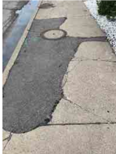
Aging pedestrian pavement along roadway requires repair. The condition of the sidewalk makes it difficult for people to walk and roll.
