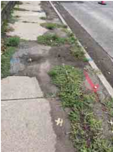
Aging pedestrian pavement along roadway requires repair. The condition of the sidewalk makes it difficult for people to walk and roll.
