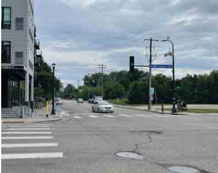
The intersection of Marshall St NE (CSAH 23) and NE Lowry Ave (CSAH 153) pictured above. Traffic signals are aging and require replacement.
