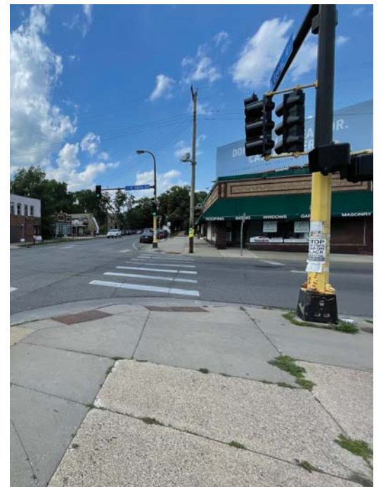
The signal system at Cedar Ave (CSAH 152) and 38th St was constructed in 1966 and will be upgraded as part of this project.
