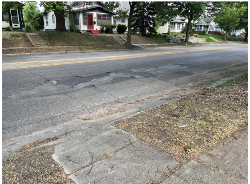
The roadway surface was last reconstructed in 1966 and requires repair.
