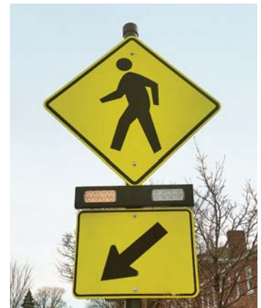
Rectangular Rapid Flashing Beacon
