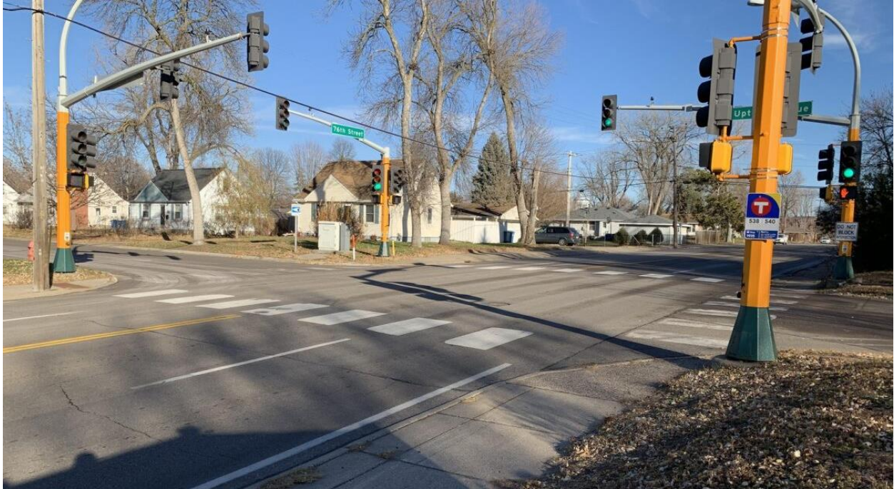
Photo 3: Existing signals at W 76th St and Upton Ave S intersection to be replaced (Nov 2023). Photo Credit: City of Richfield
