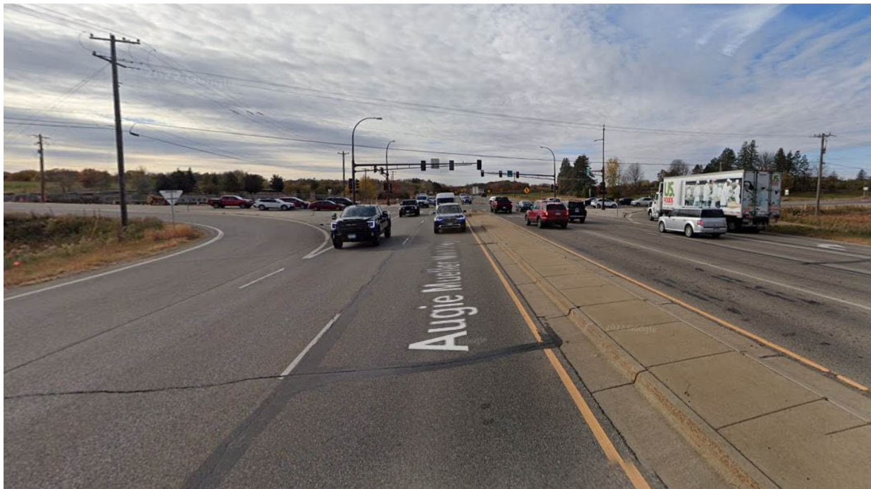
TH 5 looking east past TH 41 Intersection
