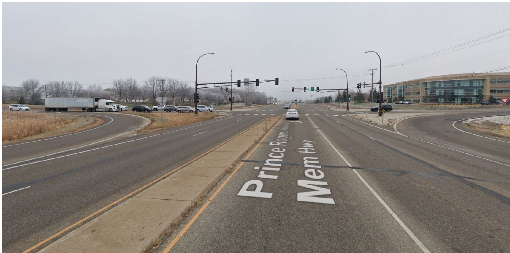
TH 5 looking east past TH 41 Intersection
