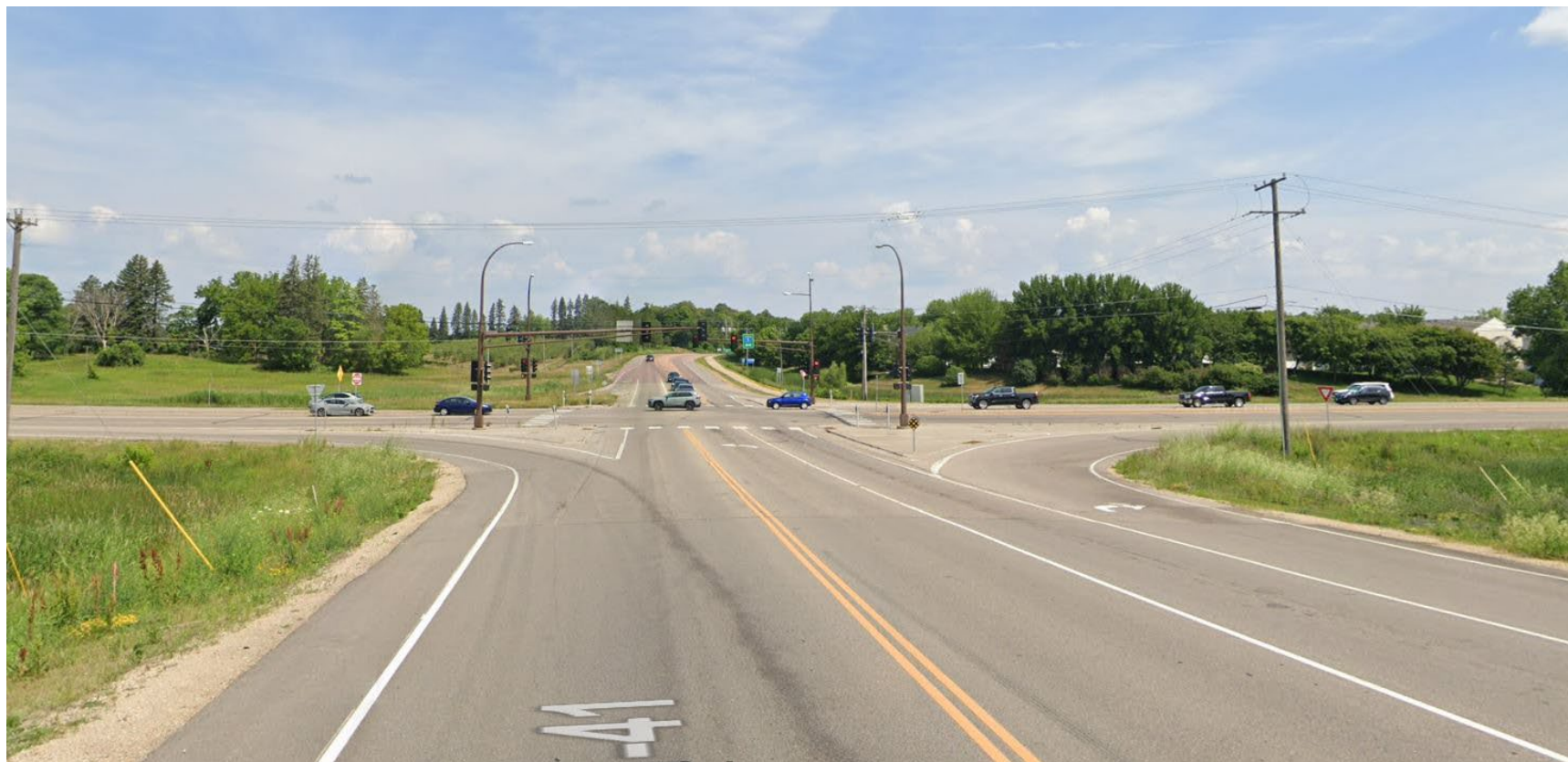
TH 41 looking north past TH 5 Intersection
