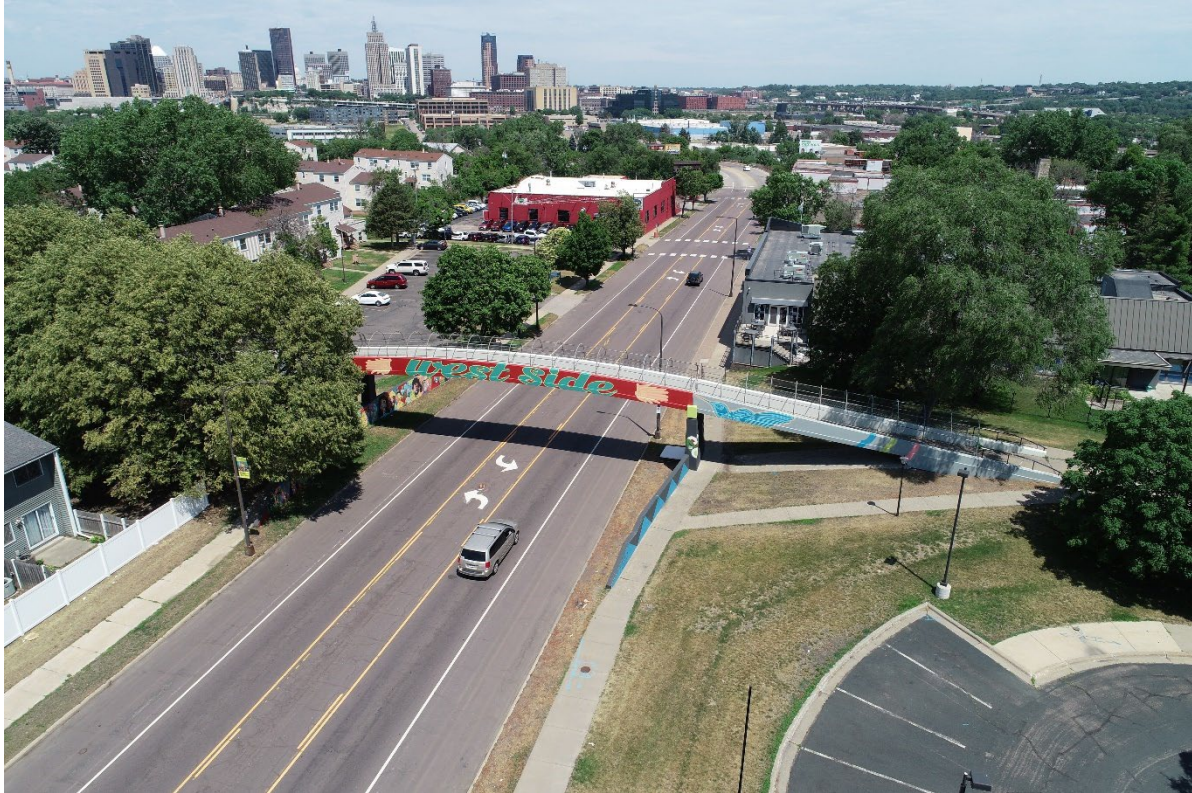
Photo: Pedestrian Bridge over Robert Street – North to the top of page.
