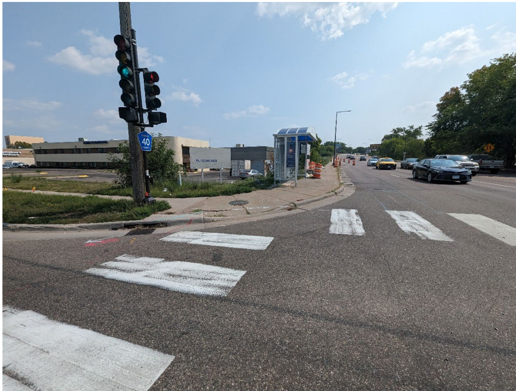
Photo: Curb ramp at Robert Street and Plato Boulevard Intersection – North to the bottom of page.
