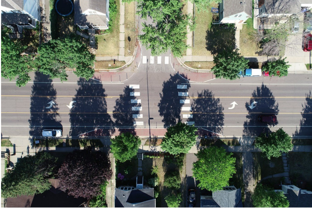
Photo: Robert Street and Baker Street Intersection – North to the Right.
