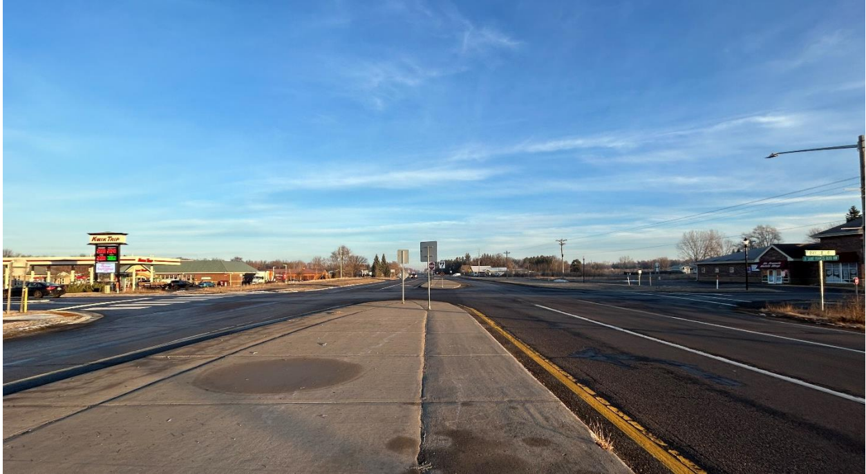
Photo 3: TH 47 at 233 rd Ave looking north (December 2023).
