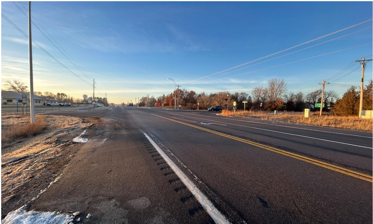
Photo 4: TH 47 at Ambassador Blvd NW looking south (December 2023).
