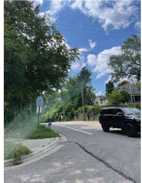
This bikeway project will include a multi-use trail to allow people to walk, bike, and roll safely.
