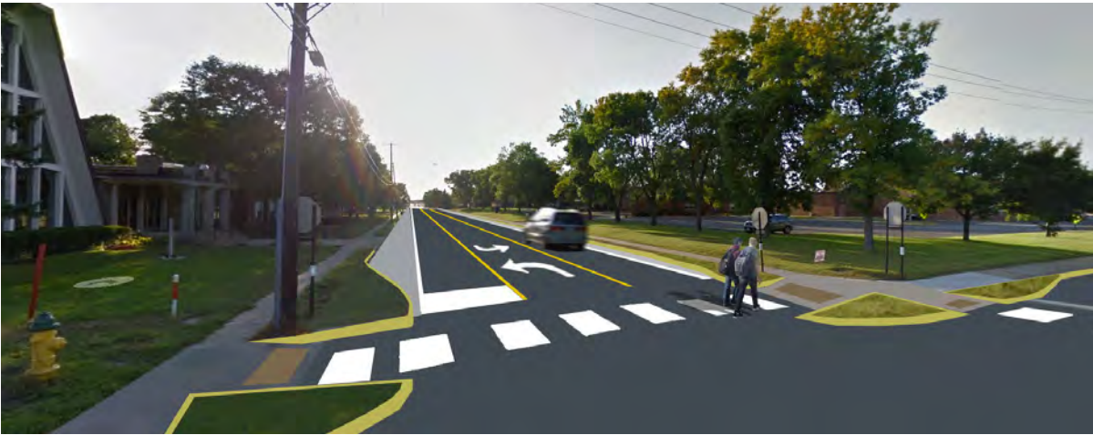
Recommendations D & F. Mississippi St NE at Monroe St NE. Current (top) and recommended (bottom). High visibility crosswalks, curb extensions and a four to three lane conversion of Mississippi St. Coordinate with County plans to implement a road diet on this corridor.
