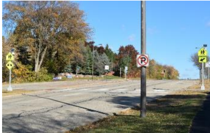
Existing school crossing on Ipava Avenue
