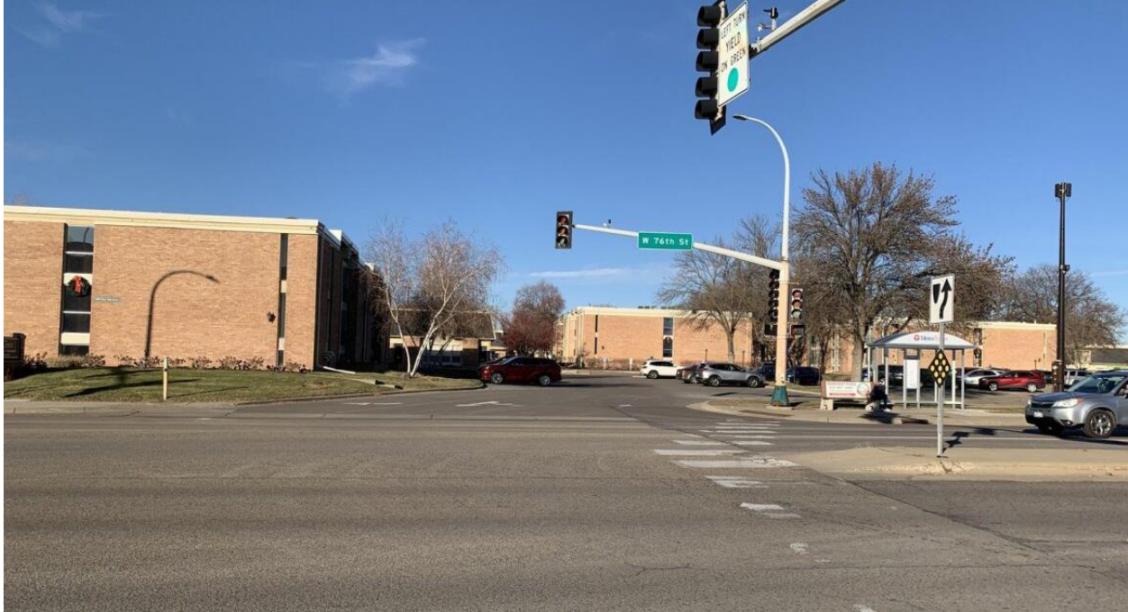
Photo 3: Looking north from southeast intersection quadrant, showing existing westbound bus stop and angled pedestrian crossing (Nov 2023). Photo Credit: City of Richfield
