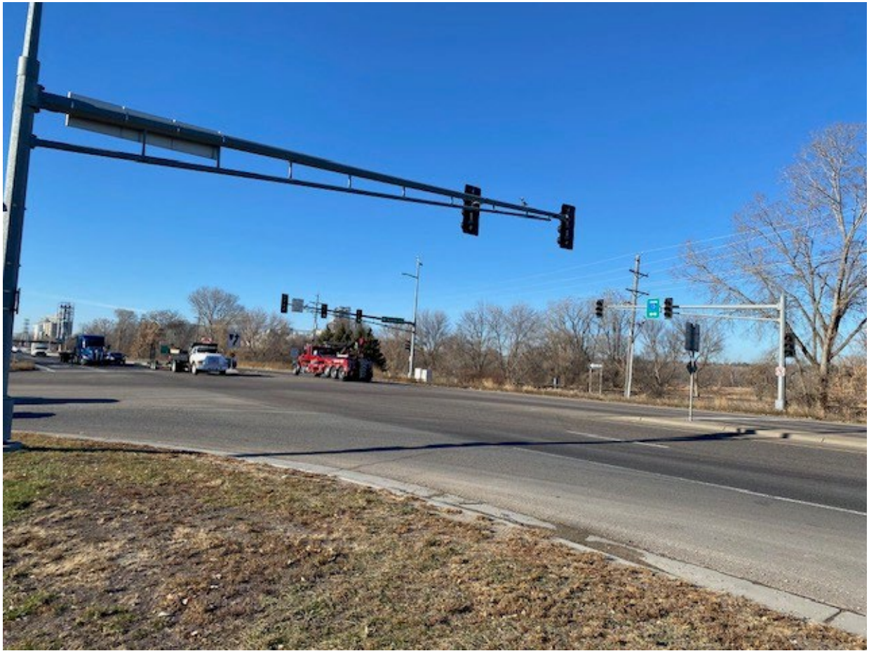
TH 13 and Quentin Avenue Intersection
