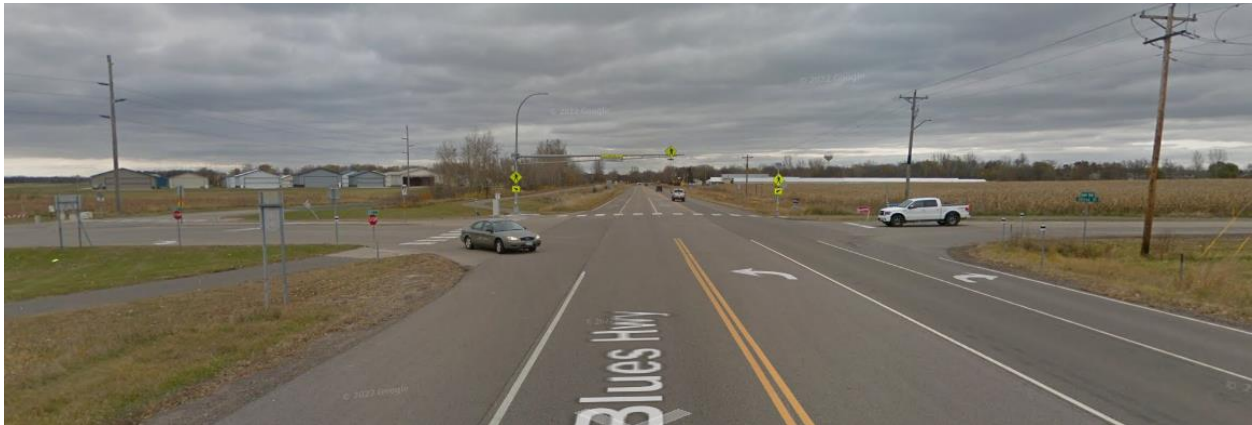
Image 2. Highway 61 at CR 50, facing north
