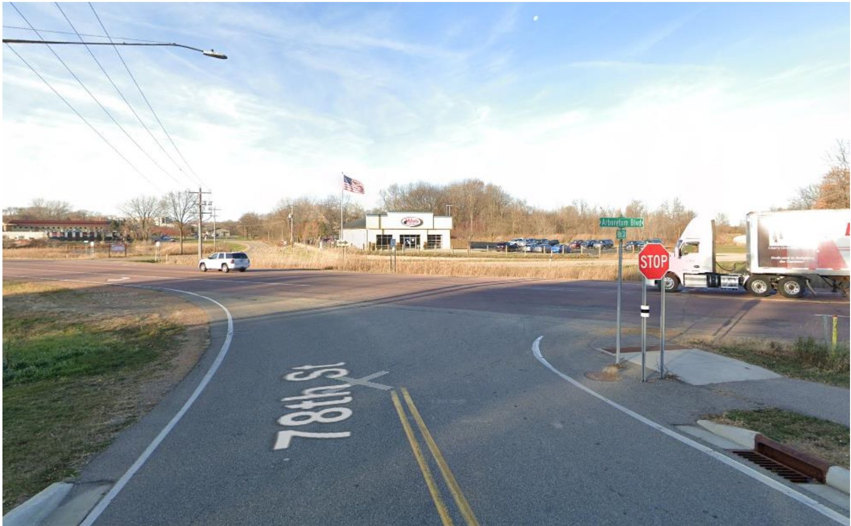
TH 5 at 78 th Street Existing Conditions – looking west
