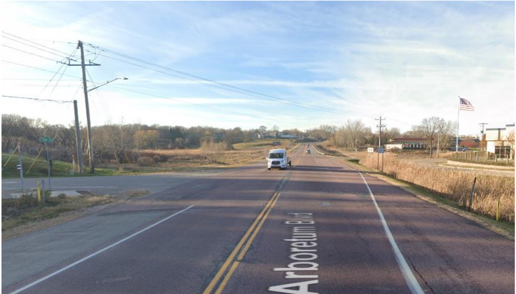
TH 5 at 78 th Street Existing Conditions – looking southwest
