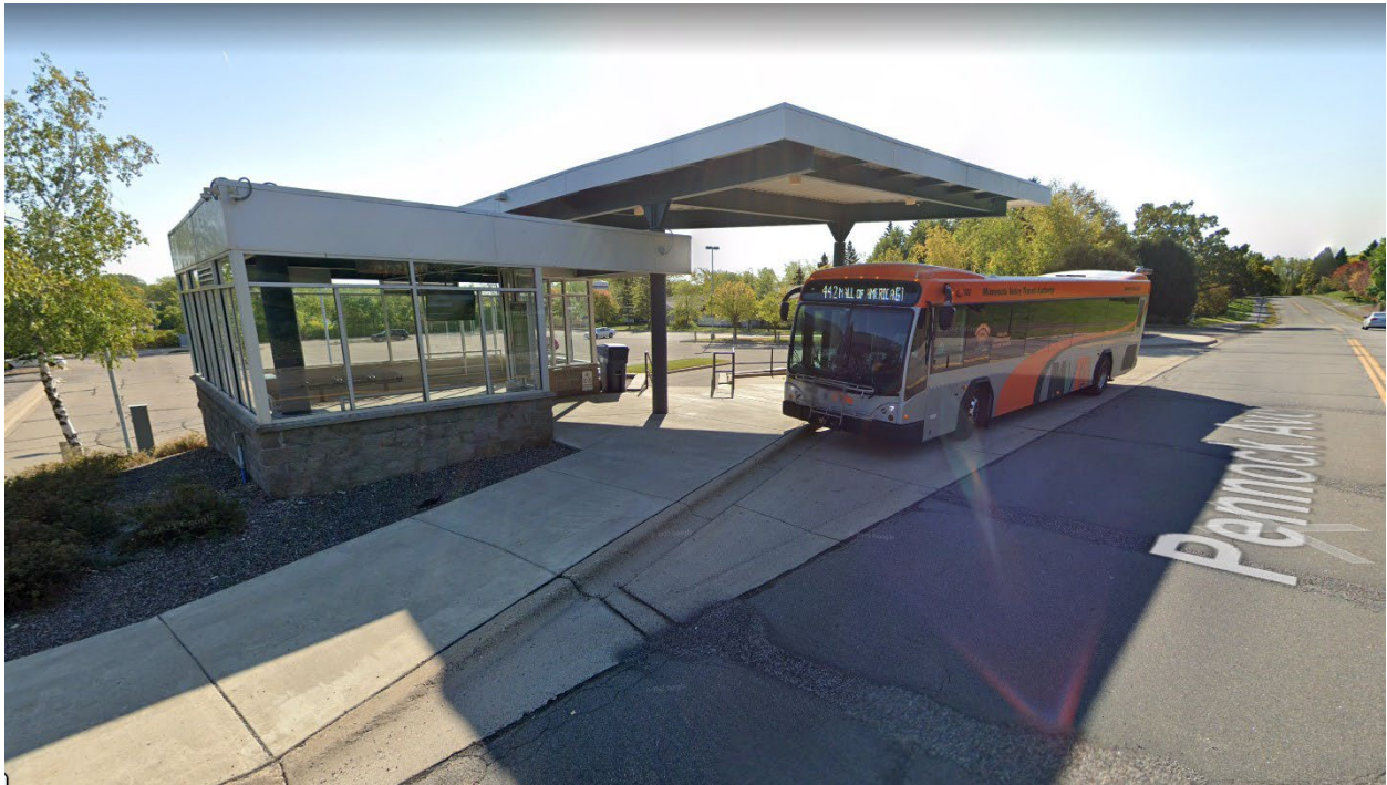
Figure 20: Street View of the Palomino Park & Ride Canopy Partially Covering the Front of a Bus
