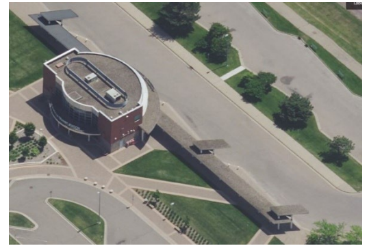
Figure 17: High/Low Canopies at Burnsville Transit Station Bus Berths
