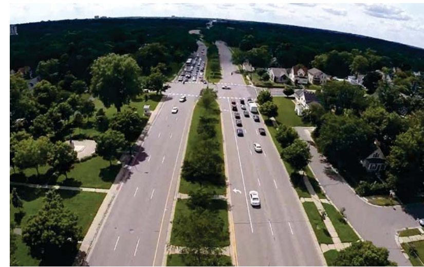
Westbound view at Penn Ave
