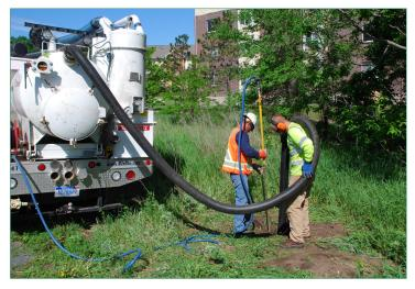
Above: Crews dig potholes in early June near Highway 100 in St. Louis Park as part of subsurface utility engineering to locate water lines for the Southwest LRT Project.
