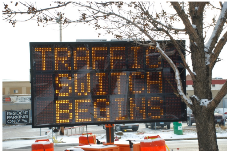
VMS used to alert drivers to the traffic switch on University Avenue
