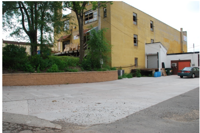
City of St. Paul Neighborhood Commercial Parking Program funds used to build a retaining wall and parking lot for Design Press at 2447 University Avenue
