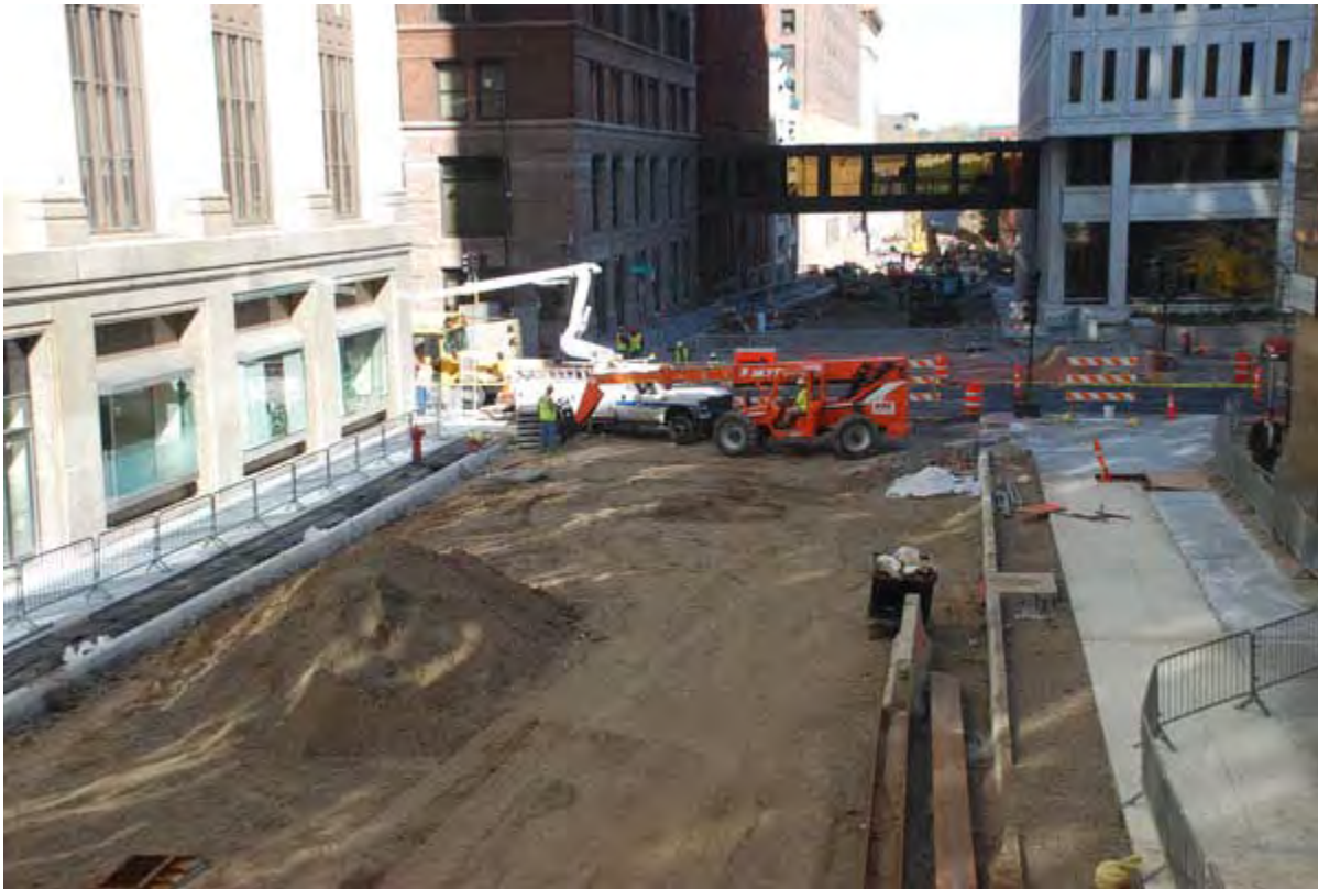
New sidewalks are being installed on Fourth Street.
