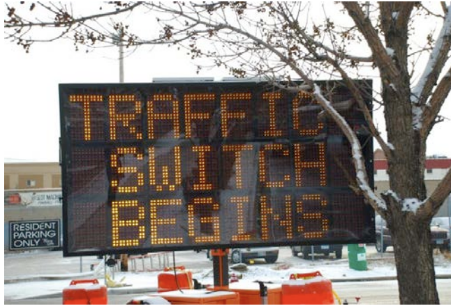
Photo 5: Variable message signing used to alert drivers to the traffic switch on University Avenue.
