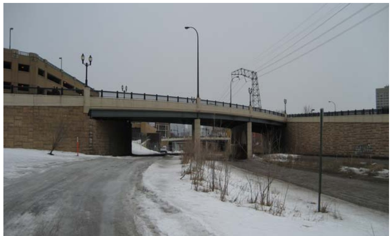
View of the proposed Northern Alignment, west toward the 5th Street SE Bridge, Dinkytown and downtown Minneapolis.
