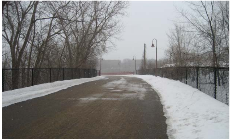
View northeast along the existing trail as it approaches Bridge No. 9 and the Mississippi River.
