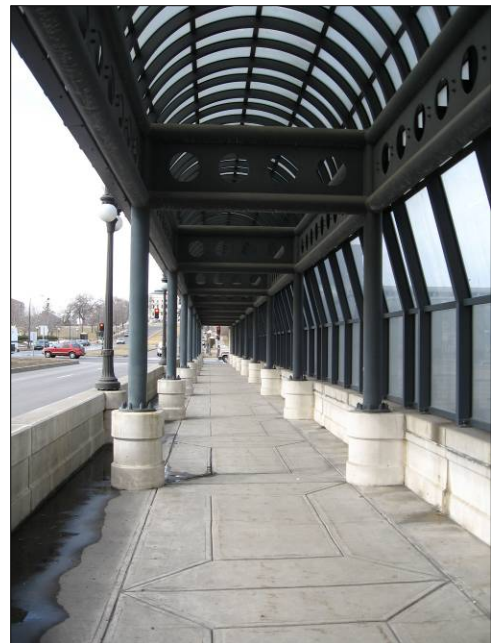
This walkway crosses I-94 between downtown St. Paul and the Capitol Area. The Central Corridor LRT would include and encourage more pedestrian-friendly facilities near LRT stations.
