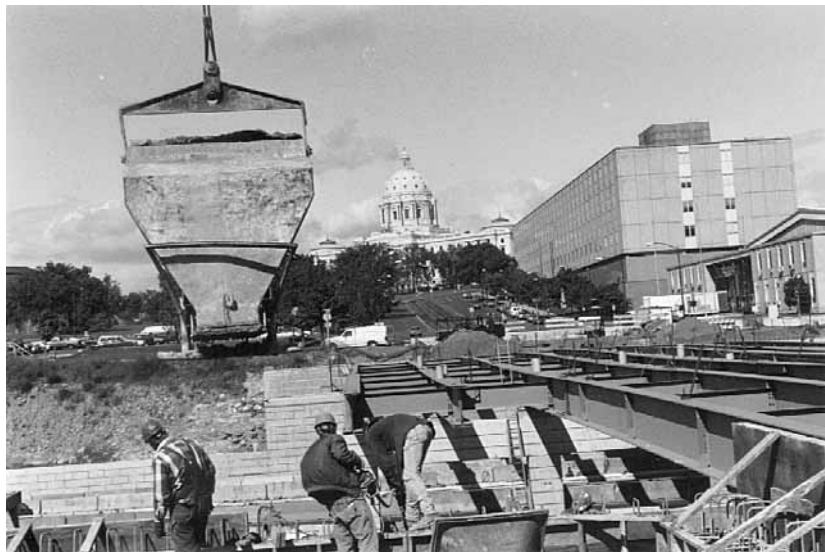
Rebuilding the Cedar Street bridge over Interstate 94 in 1992.
