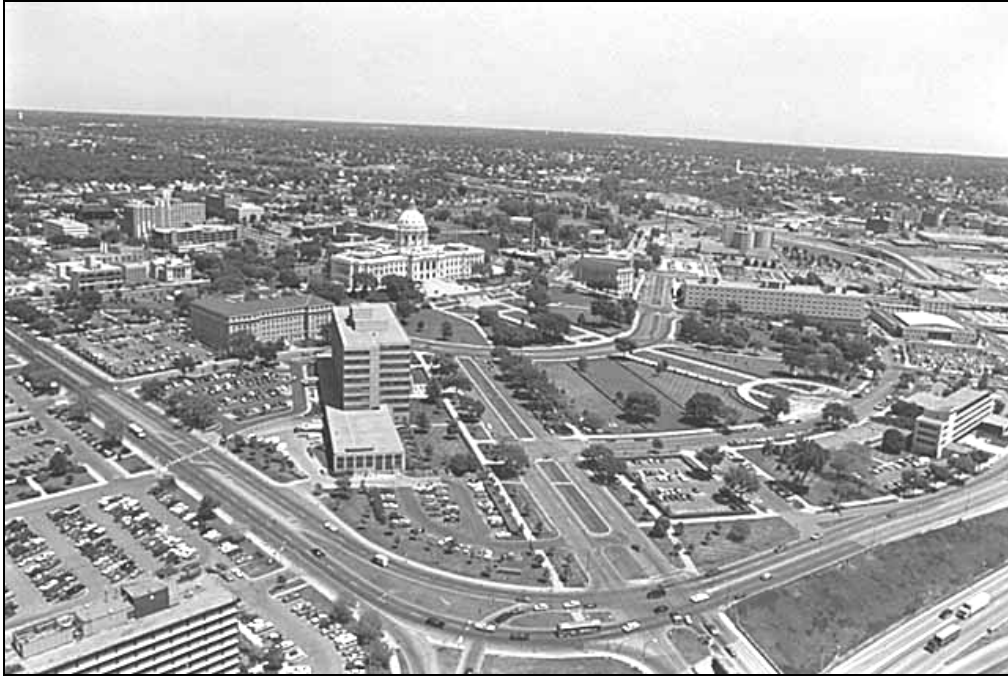
The Minnesota State Capitol Mall and Approaches in 1983 Photo: Minnesota Historical Society Collections
