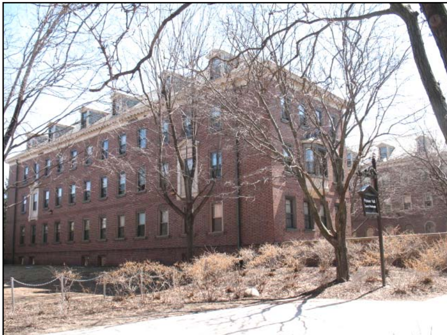
Pioneer Hall north, view from Essex Street extension
