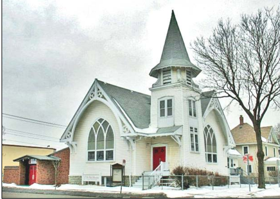
Former University Avenue Congregational Church, 507 North Victoria Street. View to southwest. Photo: Marjorie Pearson
