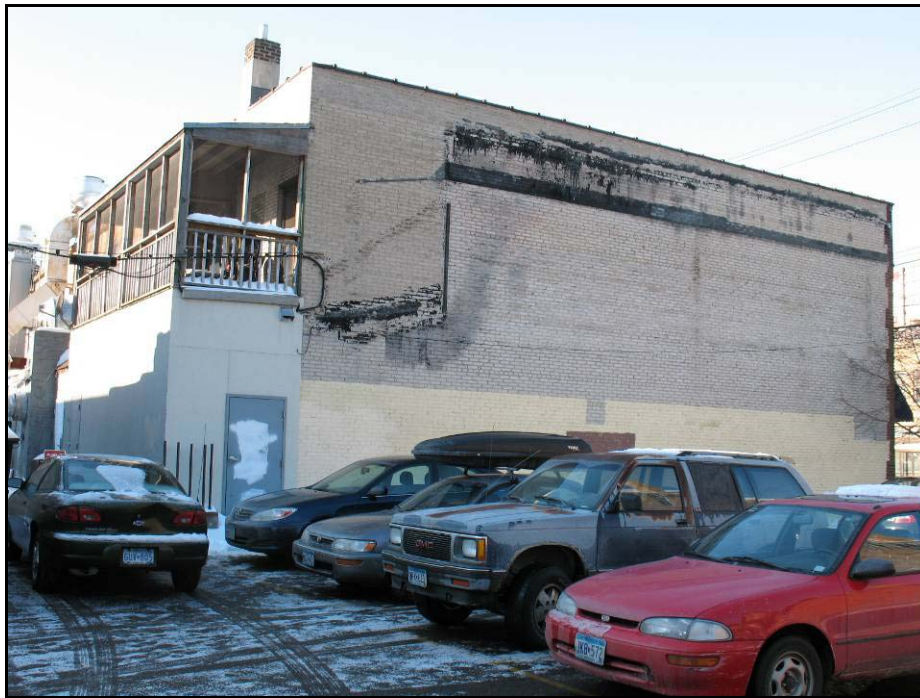
806 Washington Avenue S.E. from side and rear
