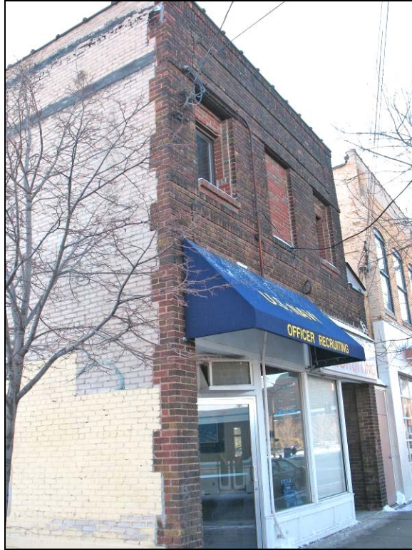
806 Washington Avenue S.E. view towards 800 Washington Avenue S.E. Photos: Penny Petersen
