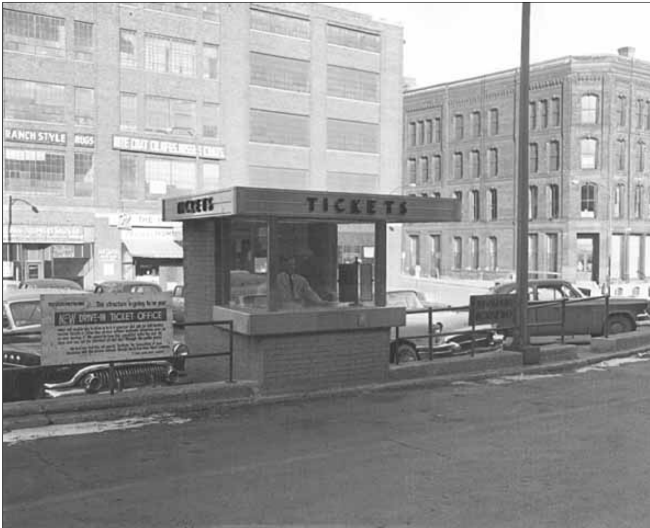
Union Depot drive-up ticket office, 1956. Note remodeled building facades along East Fourth Street behind ticket office.
