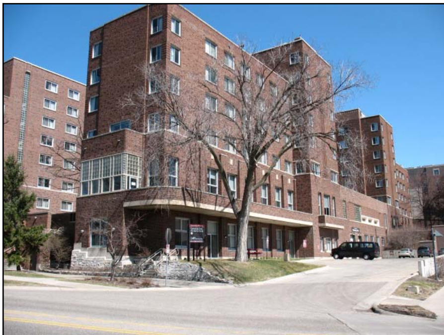
Comstock Hall from East River Parkway, view to northeast Photo: Marjorie Pearson
