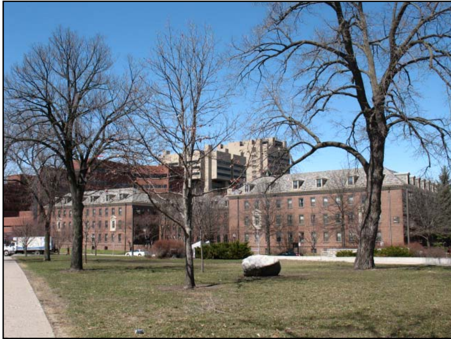
Pioneer Hall south, view from East River Parkway
