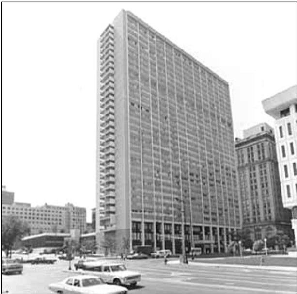
6. Kellogg Square, 111 East Kellogg Boulevard left: 1975. Photo: Minnesota Historical Society Collections below: 2008
