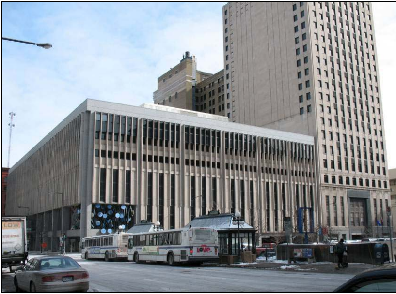
14. First Bank Addition, 332 Minnesota Street, left: 2008
