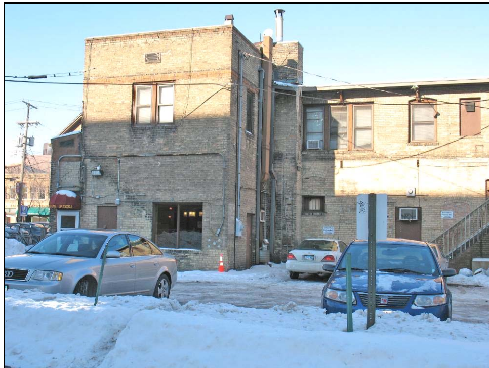
818 and 820-828 Washington Avenue S.E. from the rear
