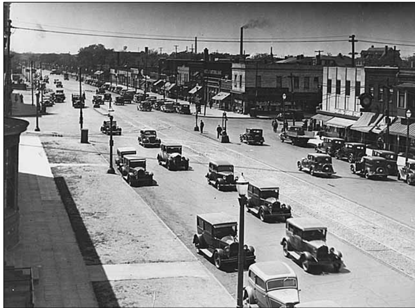
The new Walgreen's location was convenient to streetcar lines and automobile thoroughfares, as shown around 1935 in this view looking west on University towards Snelling. The Quality Park Investment Company Building is near the right edge of the photograph.
