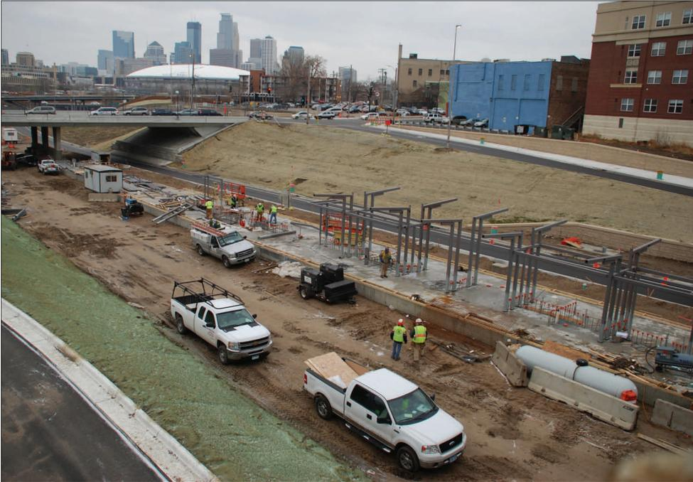
Crews erect the top of the structural steel for the West Bank Station on Washington Avenue between the Cedar and 19th avenue bridges.
