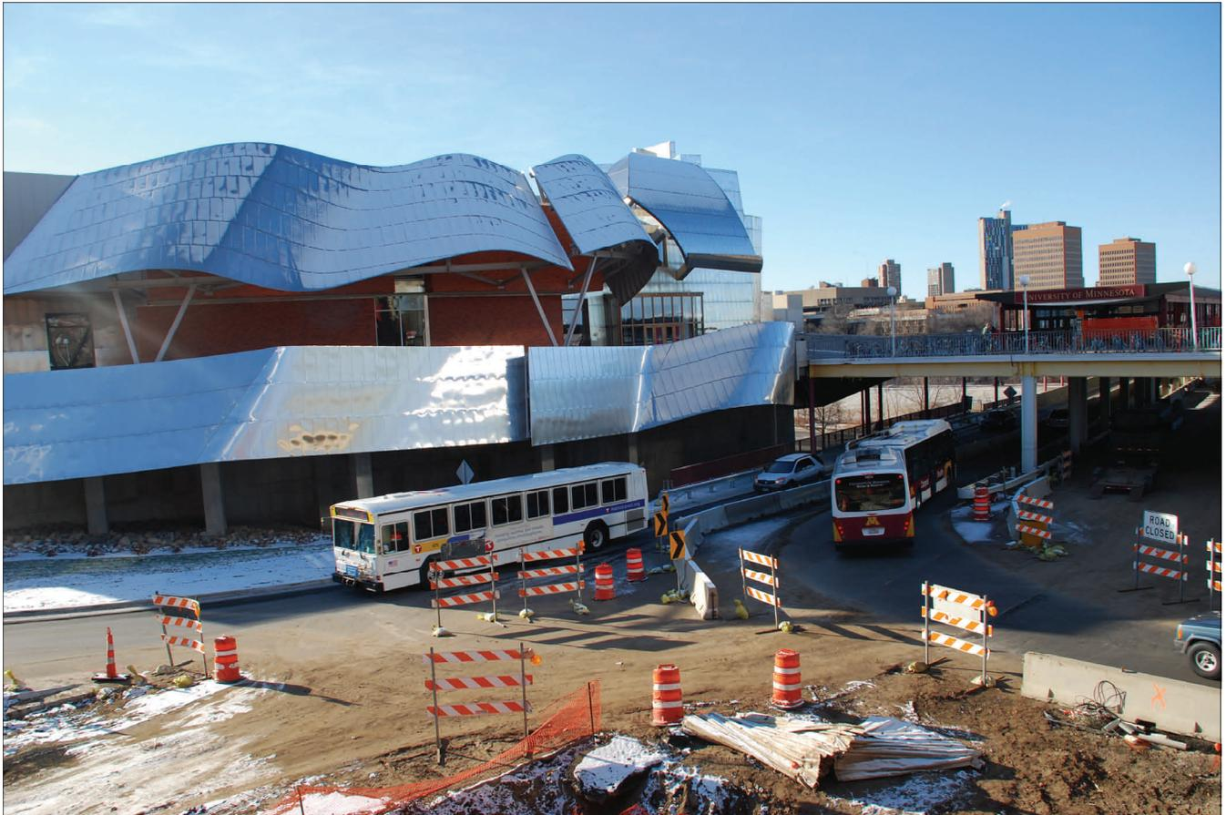
Traffic was switched in November to the newly rebuilt south side of the Washington Avenue Bridge so crews could work on the north side. Crews will work over the winter on the bridge. They are strengthening the bridge to carry light-rail trains on two tracks in the middle. In the final configuration, eastbound traffic will be single lane on the south side and westbound traffic will be single lane on the north side.
