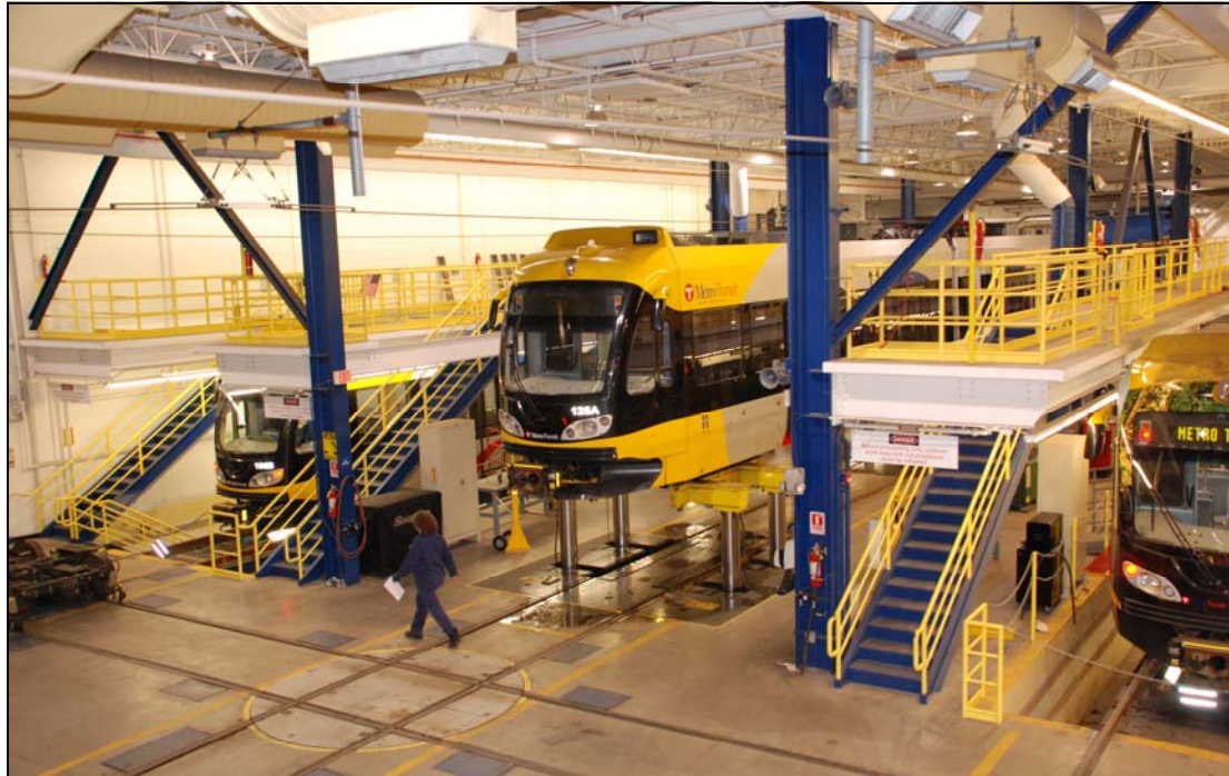
The Central Corridor LRT's operation and maintenance facility in the former Gillette Co. factory in Lowertown will resemble the Hiawatha LRT's operation and maintenance facility pictured above. Workers will clean the interior and exterior of light rail vehicles and will perform light maintenance in the enclosed facility.
