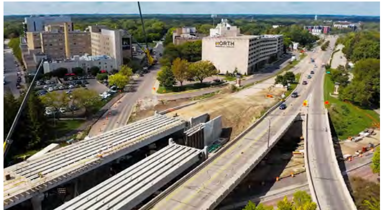
An aerial view of North Memorial
