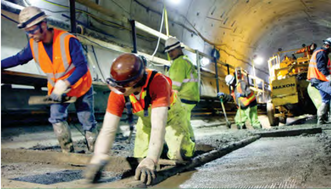
Vision of Penn Avenue Subway Construction (ref. Seattle's SoundTransit web site)
