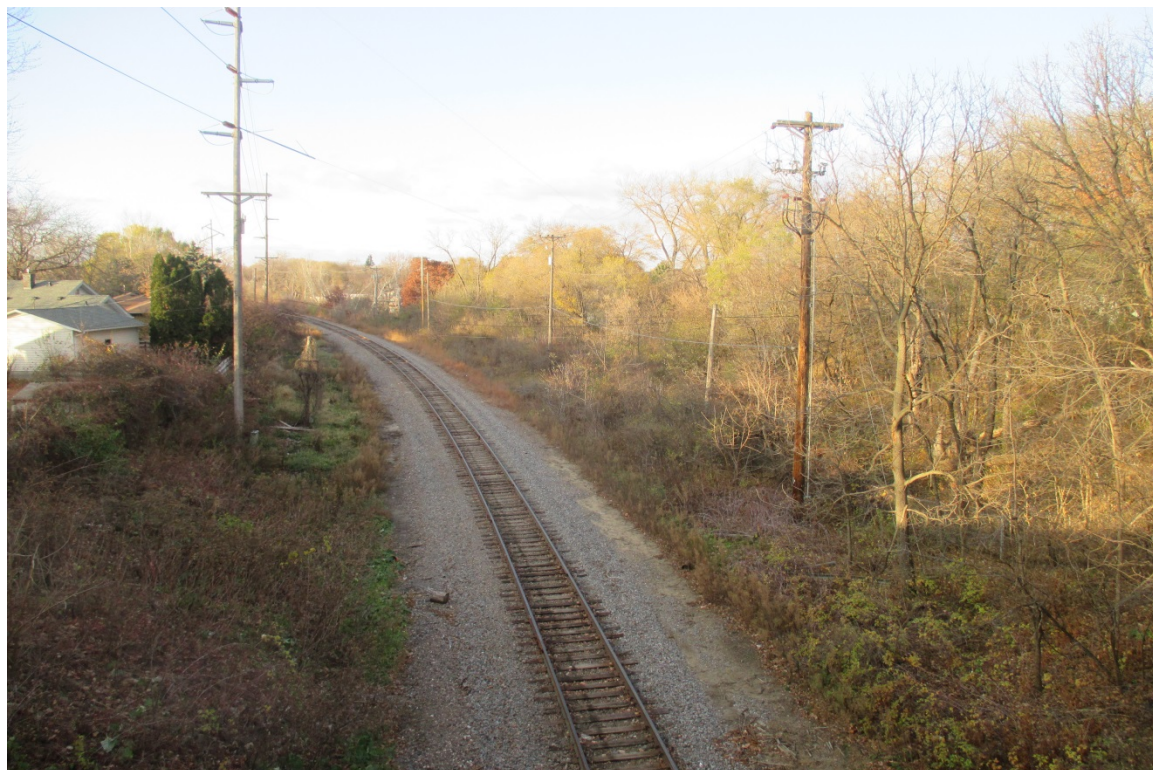
NW 2a: View to the northwest - noise walls would be on the east and west sides of the corridor
