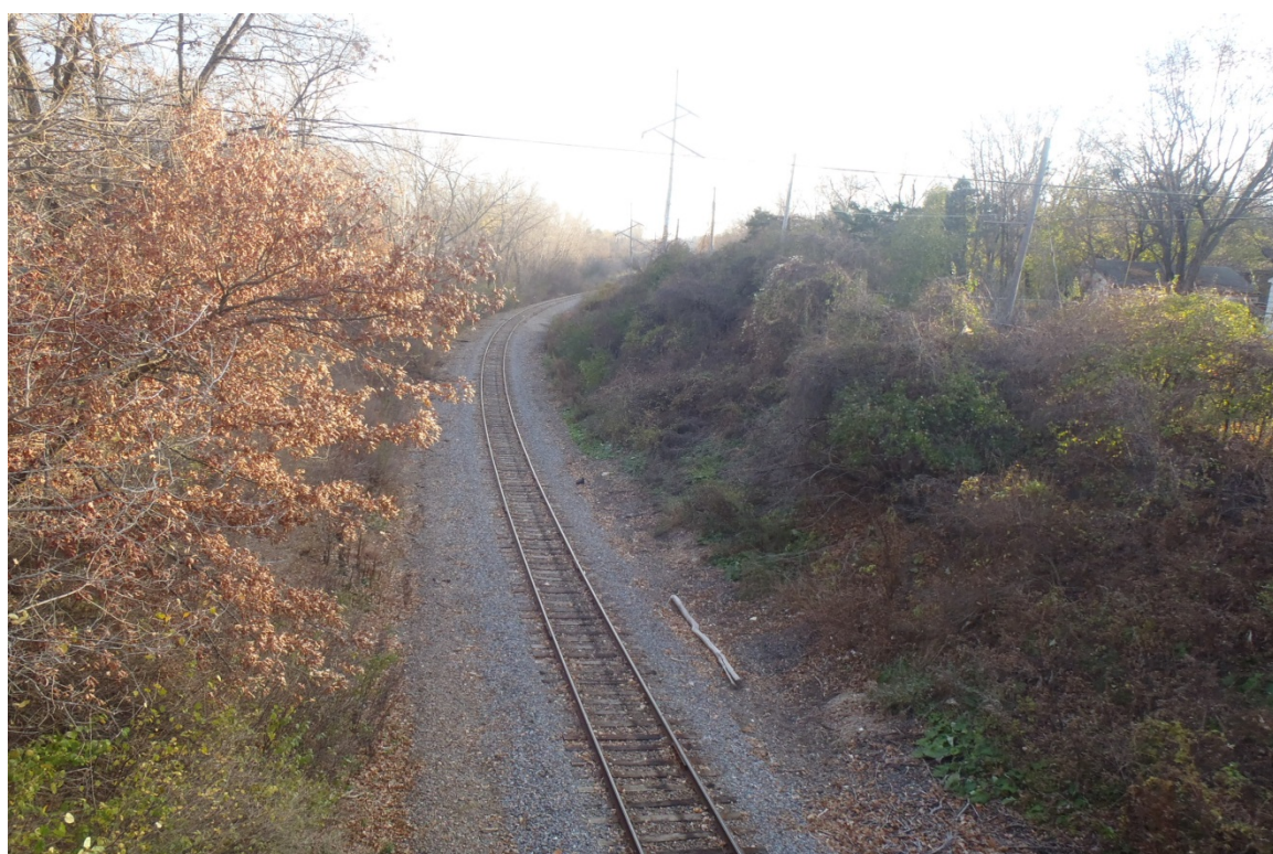
NW 2b: View to the southeast - noise wall would be on the east side of the corridor (left in the photo)
