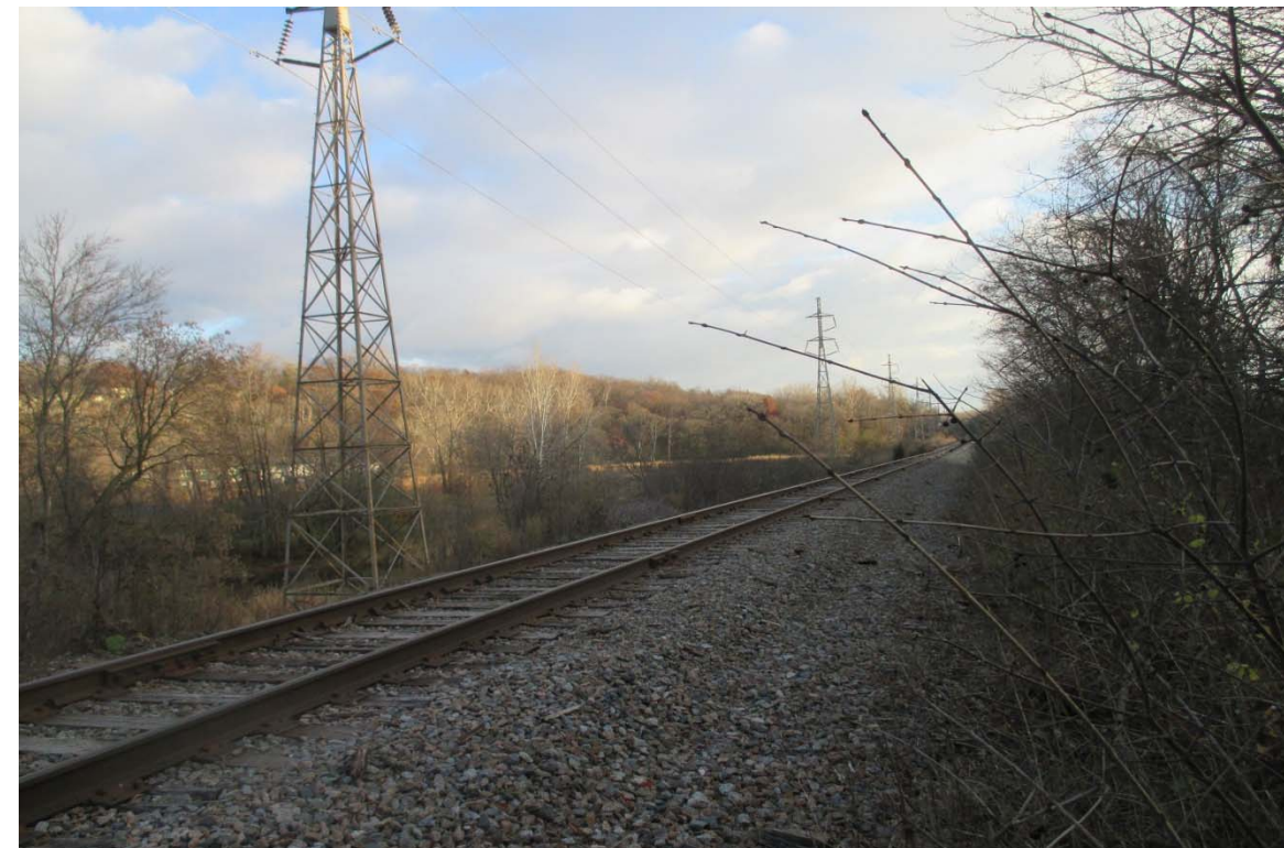
NW 1b: View to the southeast - noise wall would be on the east side in the background (left of the corridor in the photo)
