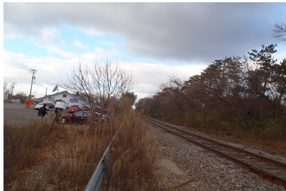
NW 3a: View to the northwest - noise wall would be on the east side of the corridor (right in the photo)
