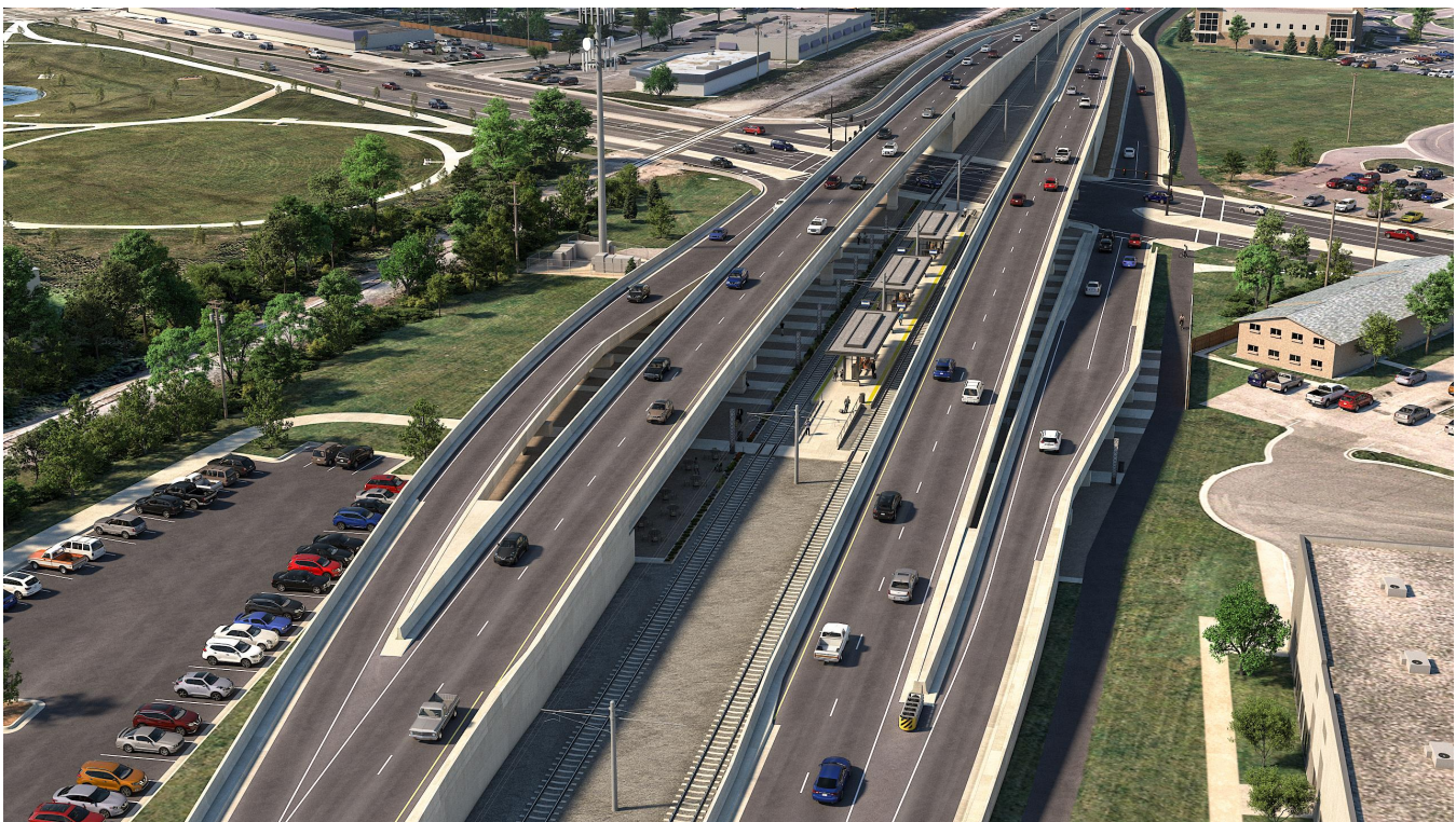
Figure 2-6 Grade-Separated Intersection at Bass Lake Rd/CR 81
