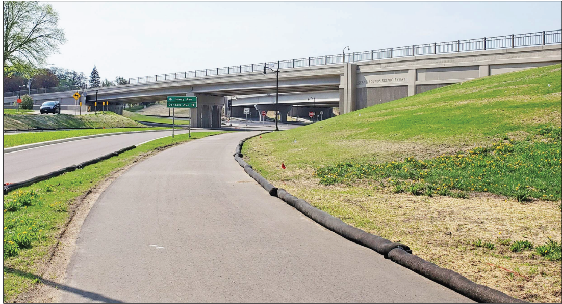
Figure 11. Current view looking south toward proposed Lowry Ave Station from Victory Memorial Drive within the Grand Rounds Historic District non-contributing segment (SEH 2025, visual renderings prepared by Kimley Horn & Associates).
