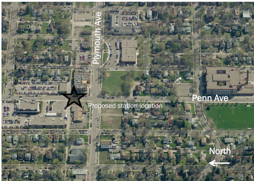
View of Penn/Plymouth intersection from the west. Community institutional uses are a focus of this neighborhood intersection.
