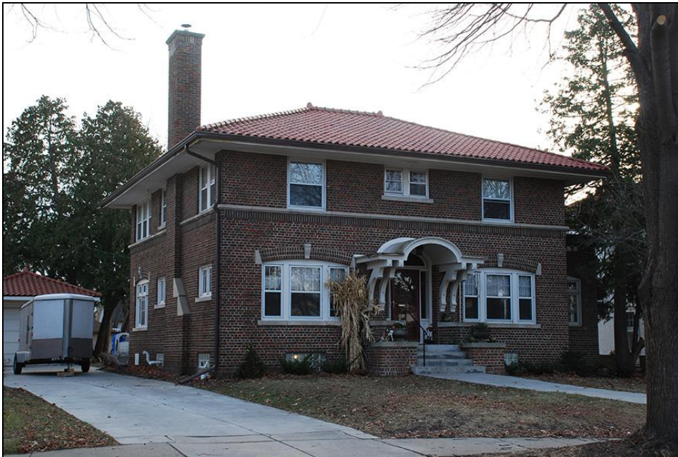
FIGURE 61. DAVID DWORSKY HOUSE (HE-MPC-7641), 2515 12 TH AVENUE NORTH, FACING SOUTHWEST
