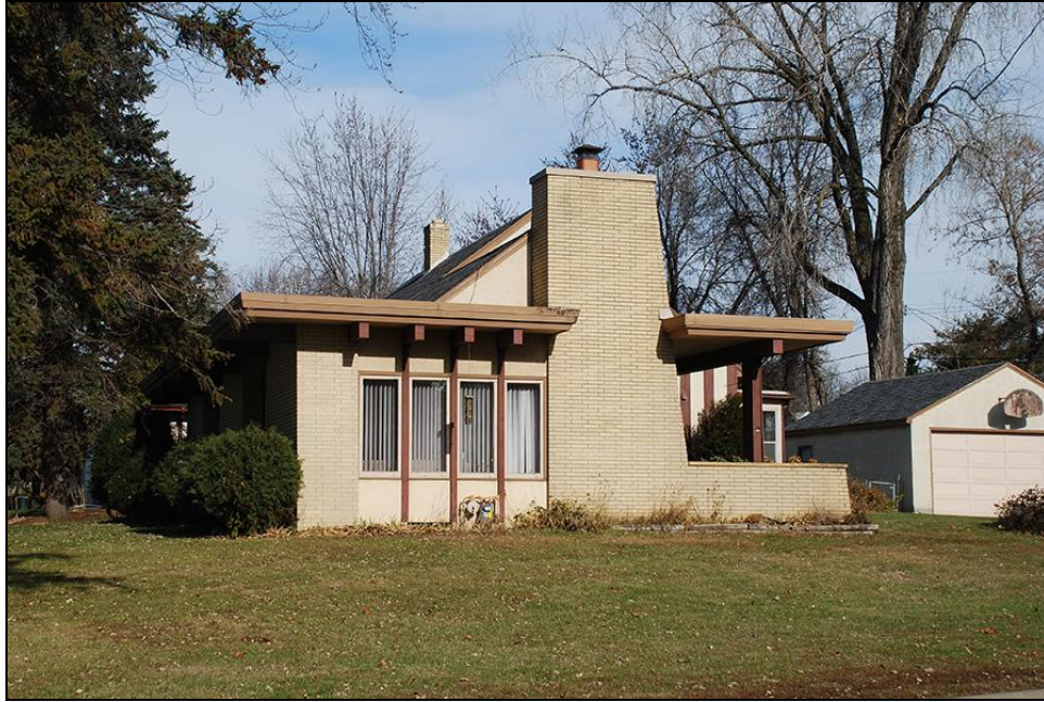
FIGURE 49. JERRY KRANZ HOUSE (HE-GVC-348). FACING NORTH
