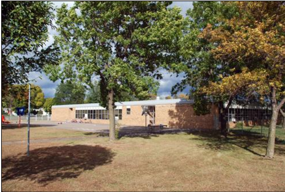
FIGURE 26. WILLIAM CAVANAGH SCHOOL (HE-CRC-100), FACING NORTHEAST
