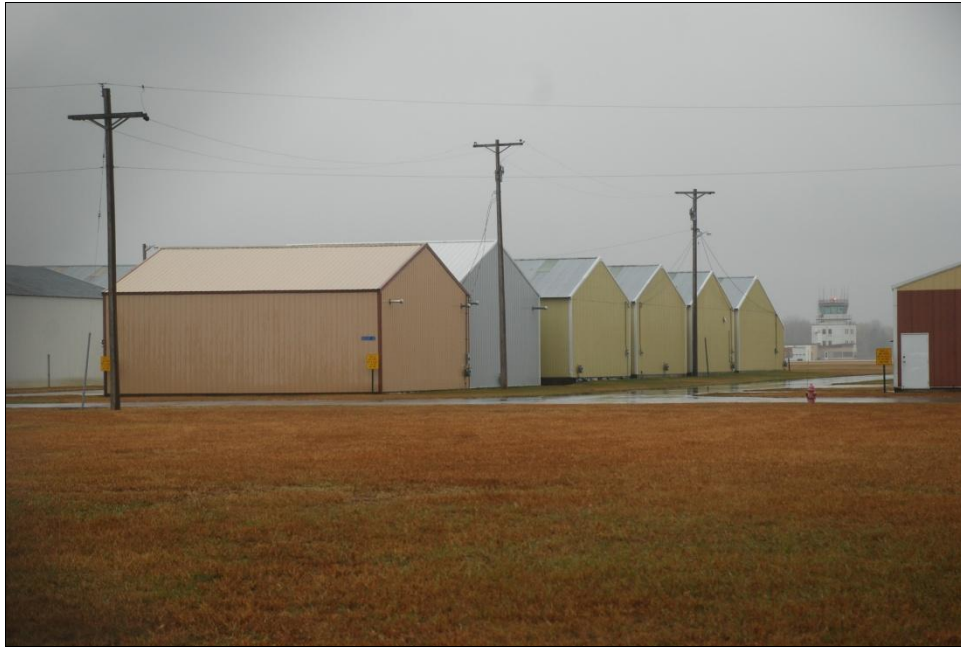
FIGURE 19. HANGARS ON THE EAST SIDE OF THE CRYSTAL AIRPORT (HE-CRC-112), FACING SOUTHWEST
