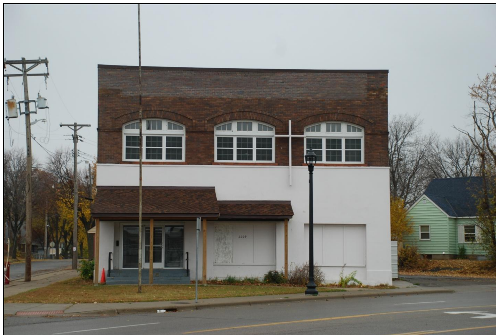
FIGURE 111. STATION 25 MINNEAPOLIS FIRE DEPARTMENT / AMERICAN LEGION NORTH SIDE POST NO. 230 (HE-MPC-8034), FACING WEST
