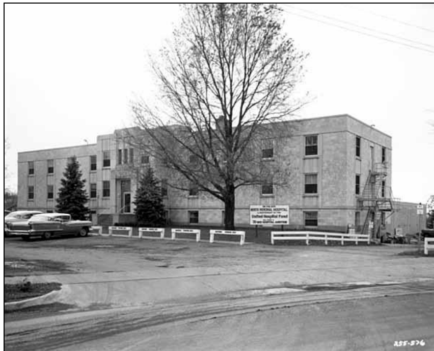
FIGURE 128. VICTORY MEMORIAL HOSPITAL / NORTH MEMORIAL HOSPITAL COMPLEX IN 1958, FACING SOUTHWEST (NORTON & PEEL 1958C)
