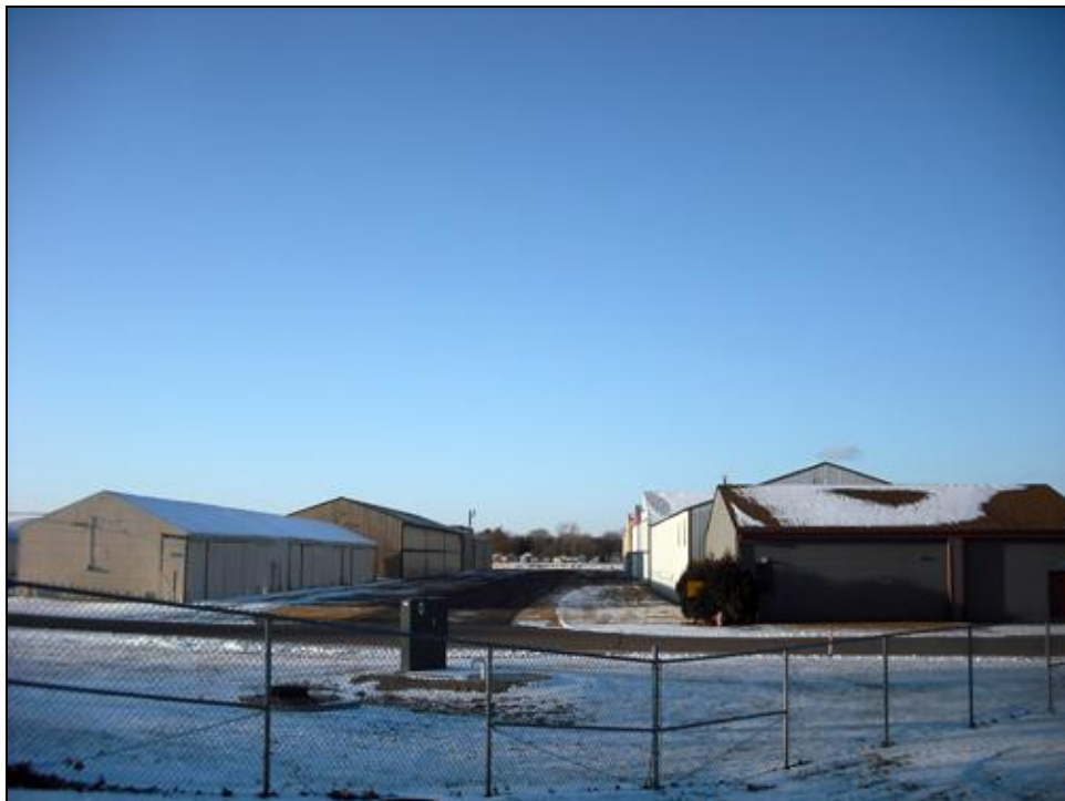
FIGURE 18. HANGARS ON THE EAST SIDE OF THE CRYSTAL AIRPORT (HE-CRC-112), FACING NORTHWEST
