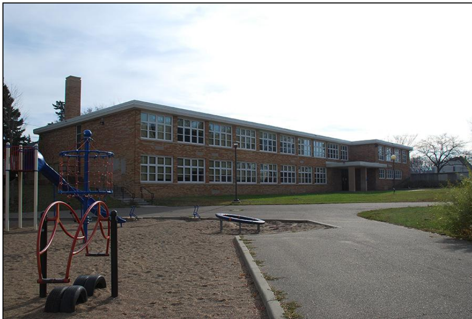
FIGURE 101. TALMUD TORAH (HE-MPC-7612), FACING SOUTHEAST
