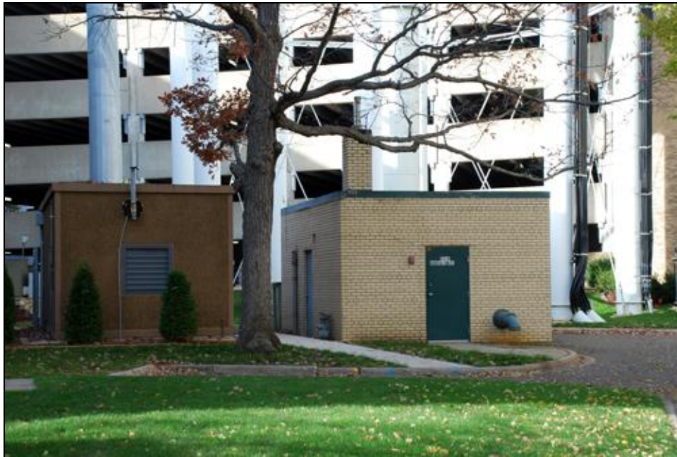
FIGURE 130. WATER TOWER NO. 2, WELL NO. 3 & FILTRATION PLANT (PUMP HOUSE AND FILTRATION PLANT) (HE-RBC-1280), FACING NORTHWEST
