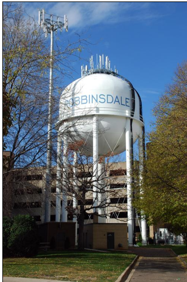
FIGURE 129. WATER TOWER NO. 2, WELL NO. 3 & FILTRATION PLANT (HE-RBC-1280), FACING NORTHWEST
