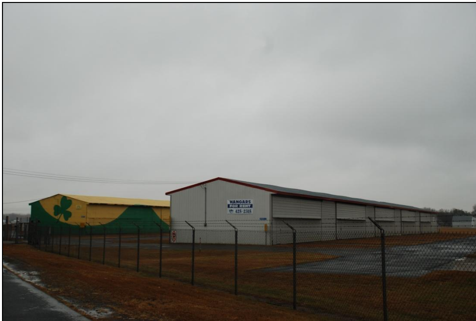
FIGURE 16. HANGARS IN THE 60 TH STREET AREA OF THE CRYSTAL AIRPORT (HE-CRC-112), FACING SOUTHEAST
