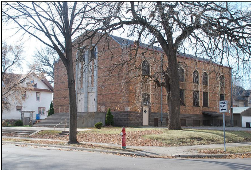
FIGURE 84. SHAREI ZEDECK SYNAGOGUE (HE-MPC-8211), FACING SOUTHWEST
