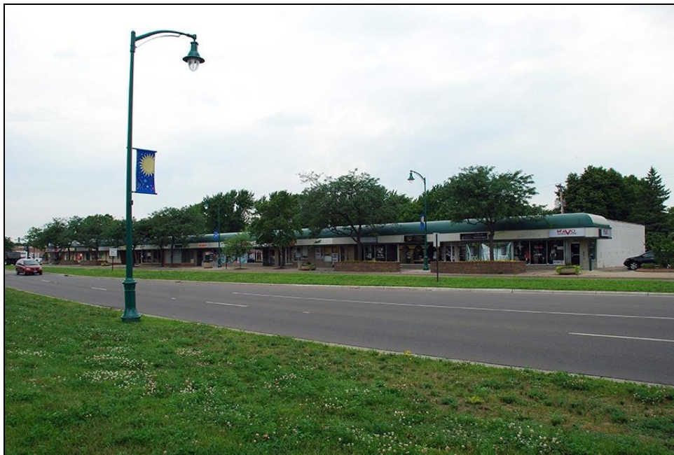
FIGURE 24. BASS LAKE ROAD COMMERCIAL AREA (HE-CRC-736), FACING NORTHWEST
