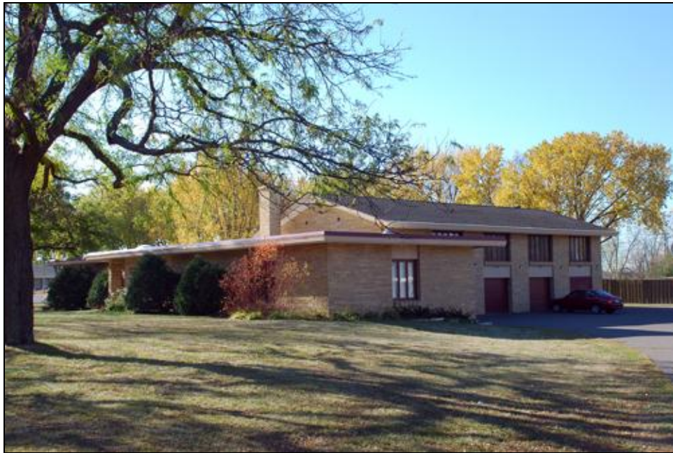
FIGURE 55. ST. MARGARET MARY RECTORY (HE-GVC-366), FACING SOUTHWEST
