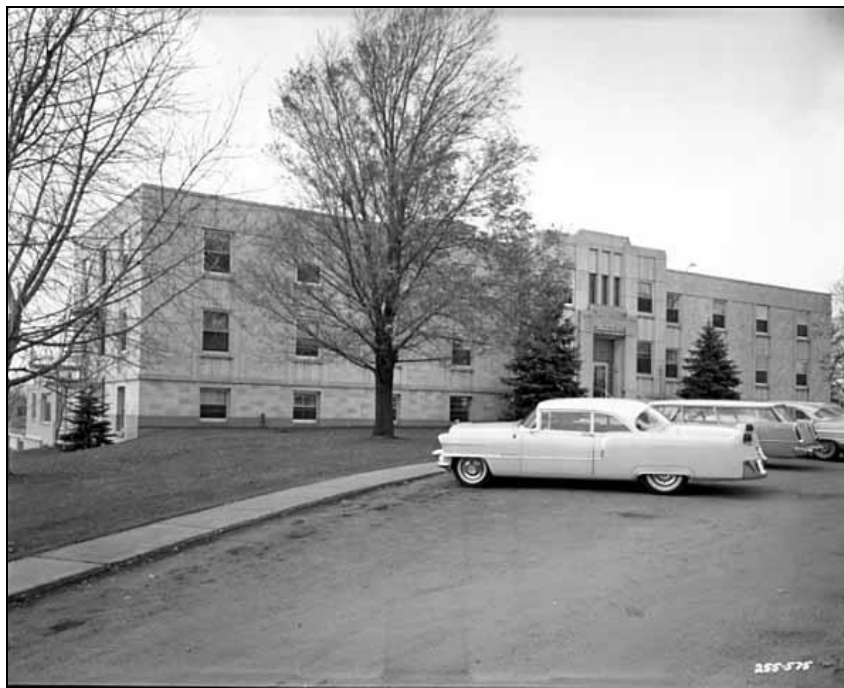
FIGURE 126. VICTORY MEMORIAL HOSPITAL / NORTH MEMORIAL HOSPITAL COMPLEX IN 1958, FACING NORTHWEST (NORTON & PEEL 1958B)
