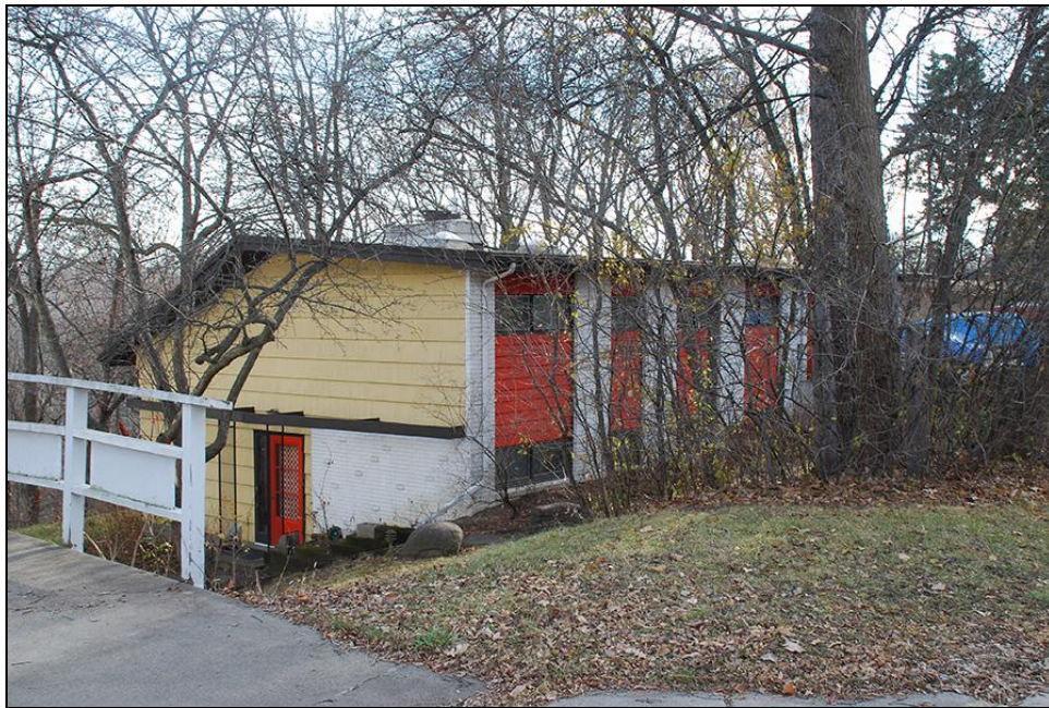
FIGURE 36. MILON GREVICH / LAWRENCE AND MARY JOHNSON HOUSE (HE-GVC-242), FACING SOUTHEAST
