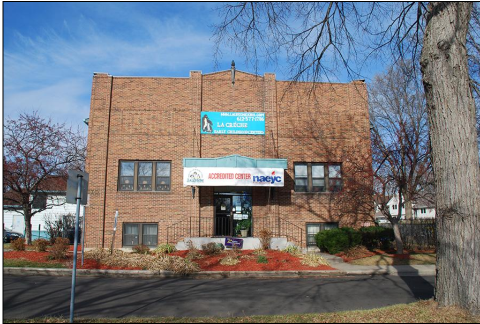
FIGURE 87. 1800 OLSON MEMORIAL HIGHWAY, HE-MPC-7553, FACING NORTH
