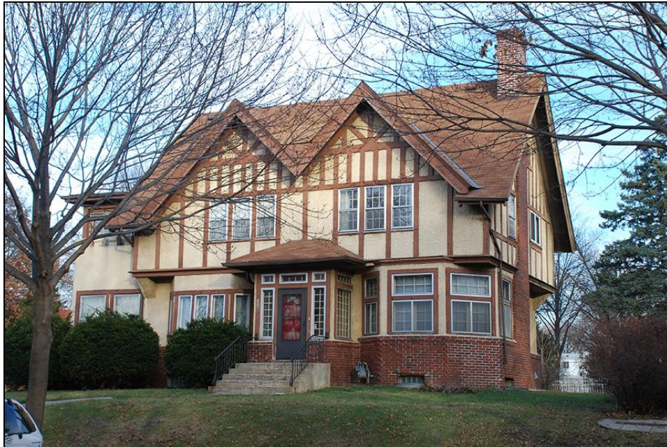
FIGURE 62. HOUSE (HE-MPC-11411), 1128 SHERIDAN AVENUE NORTH, FACING SOUTHEAST
