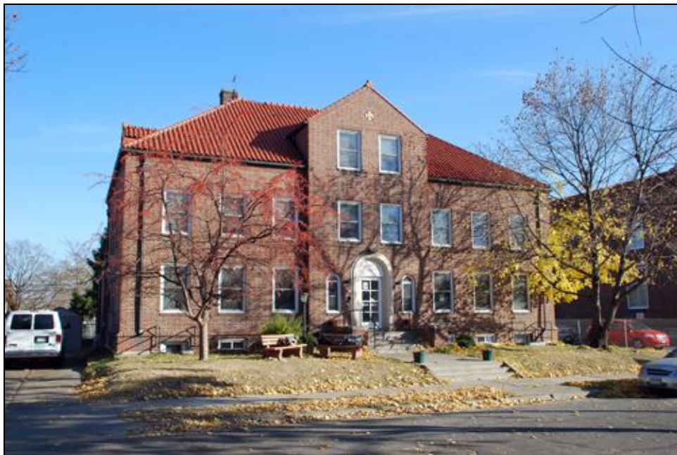
FIGURE 75. ST. ANNE'S CONVENT (HE-MPC-7505), FACING EAST
