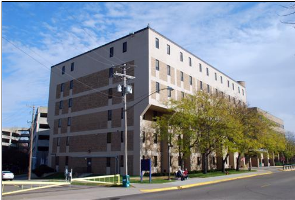
FIGURE 131. OAKDALE MEDICAL CENTER (HE-RBC-1281), FACING NORTHEAST
