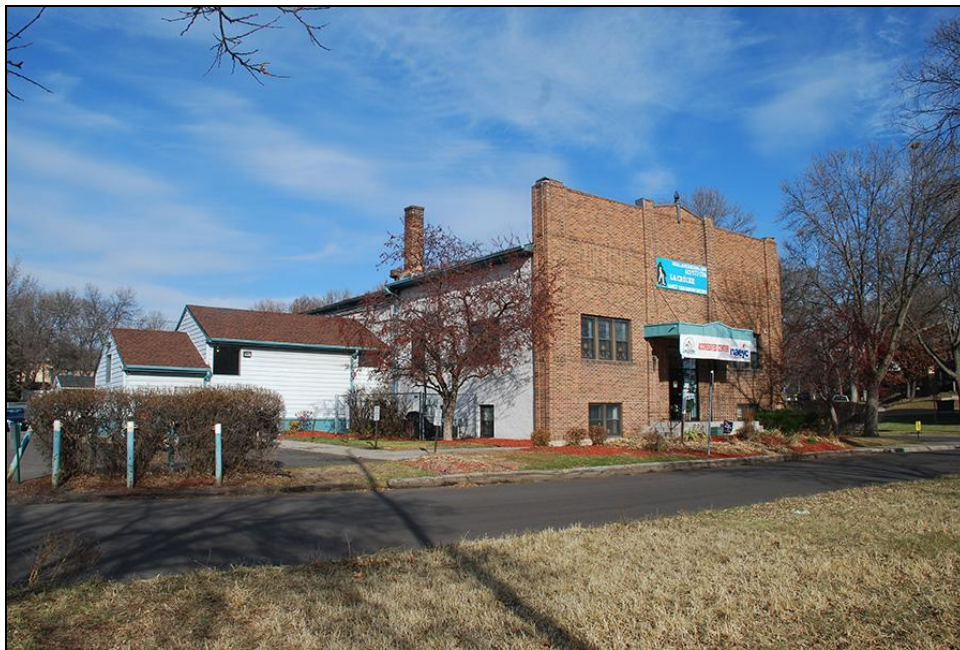
FIGURE 86. 1800 OLSON MEMORIAL HIGHWAY, HE-MPC-7553, FACING NORTHEAST
