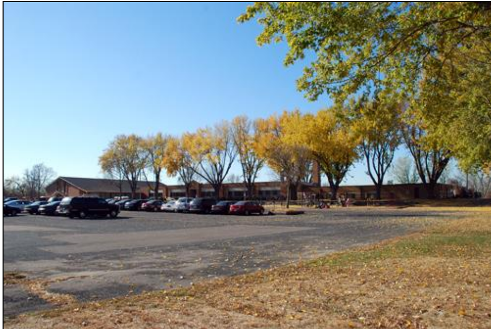
FIGURE 52. ST. MARGARET MARY CATHOLIC CHURCH & SCHOOL (HE-GVC-364), FACING SOUTHWEST
