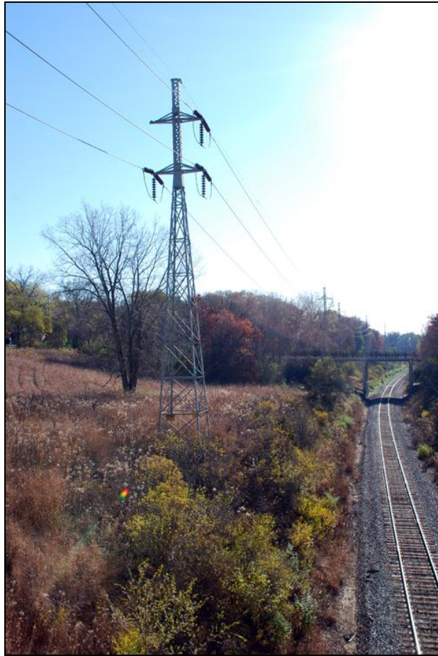
FIGURE 8. NORTHERN STATES POWER COMPANY TRANSMISSION LINE (HE-TRL-001), FACING SOUTHEAST
