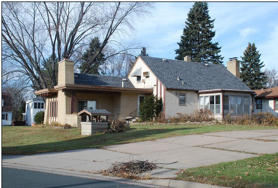
FIGURE 48. JERRY KRANZ HOUSE (HE-GVC-348), FACING NORTHEAST
