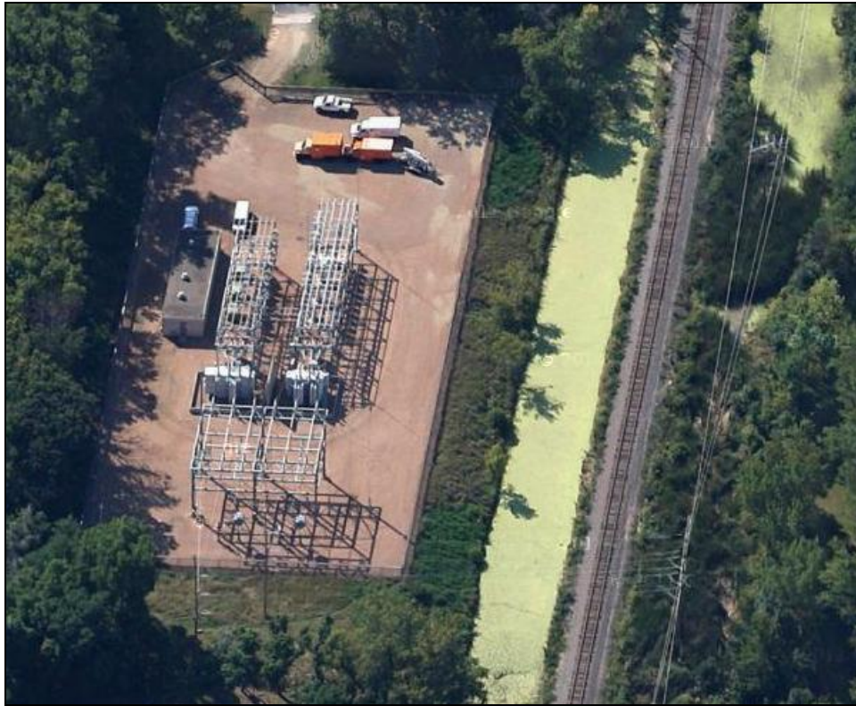
FIGURE 9. NSP SUBSTATION (HE-RBC-1264), FACING SOUTH
