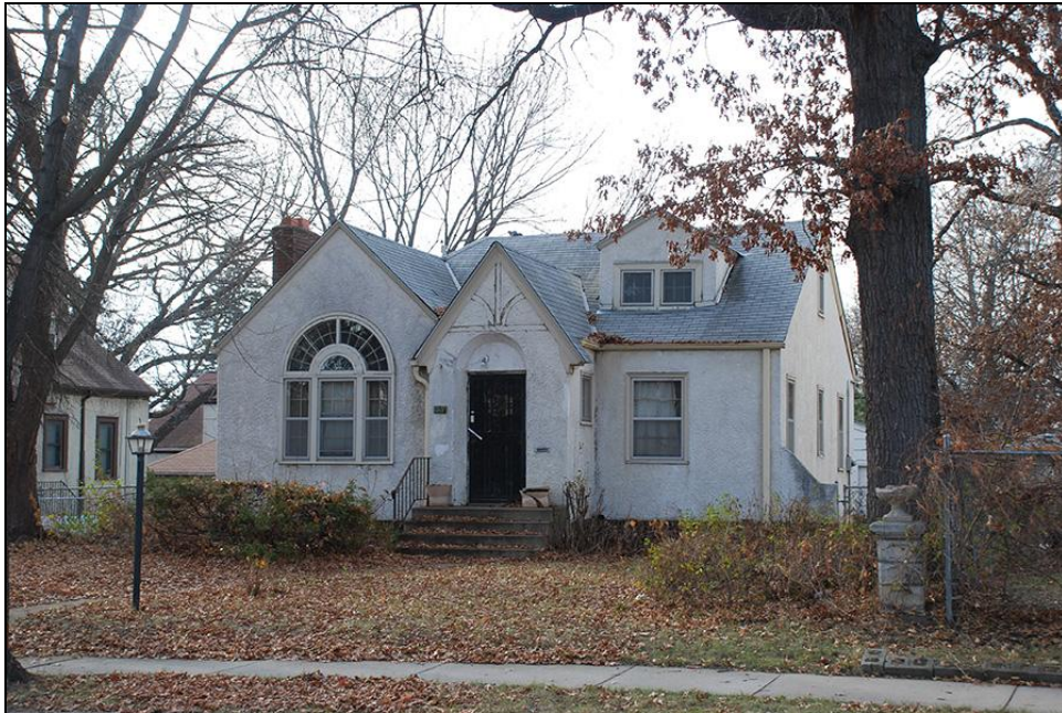
FIGURE 60. HOUSE (HE-MPC-11266), 1107 RUSSELL AVENUE NORTH, FACING SOUTHWEST
