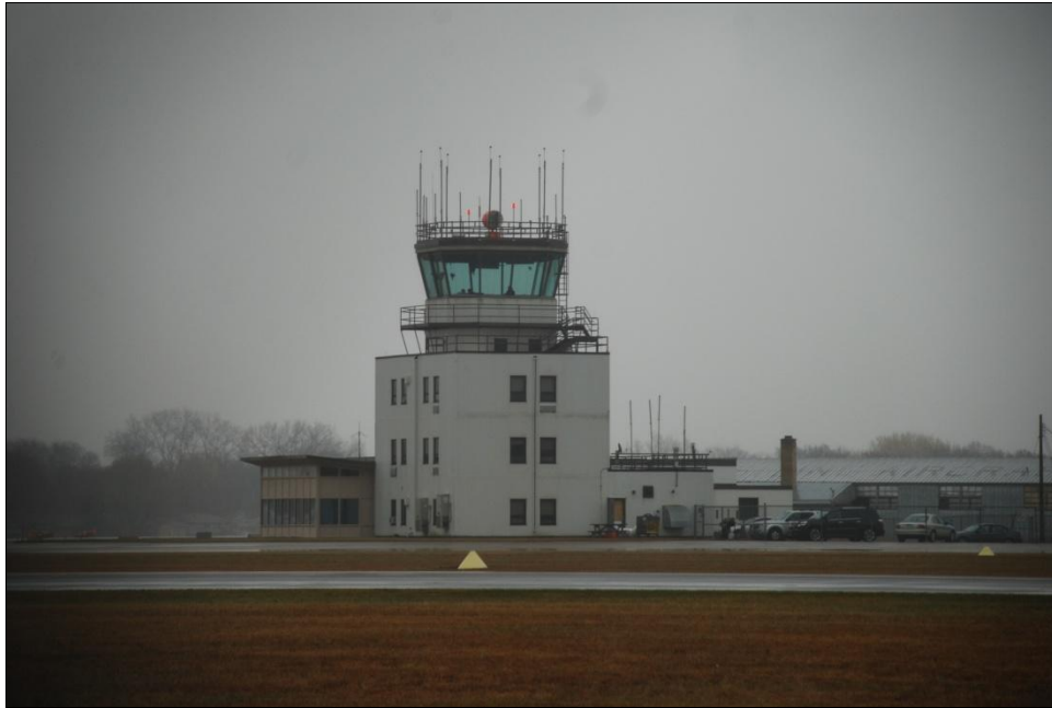
FIGURE 15. CONTROL TOWER, CRYSTAL AIRPORT (HE-CRC-112), FACING SOUTHEAST
