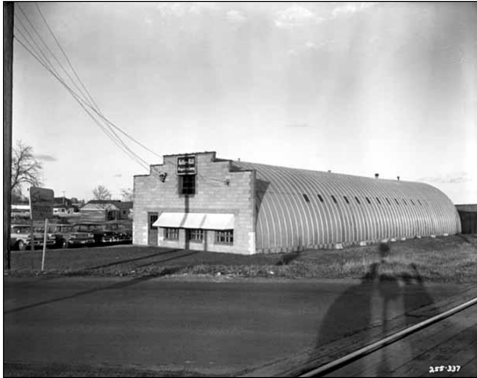
FIGURE 32. BETTER BILT MANUFACTURING IN 1958, FACING NORTHEAST (NORTON & PEEL 1958A)
