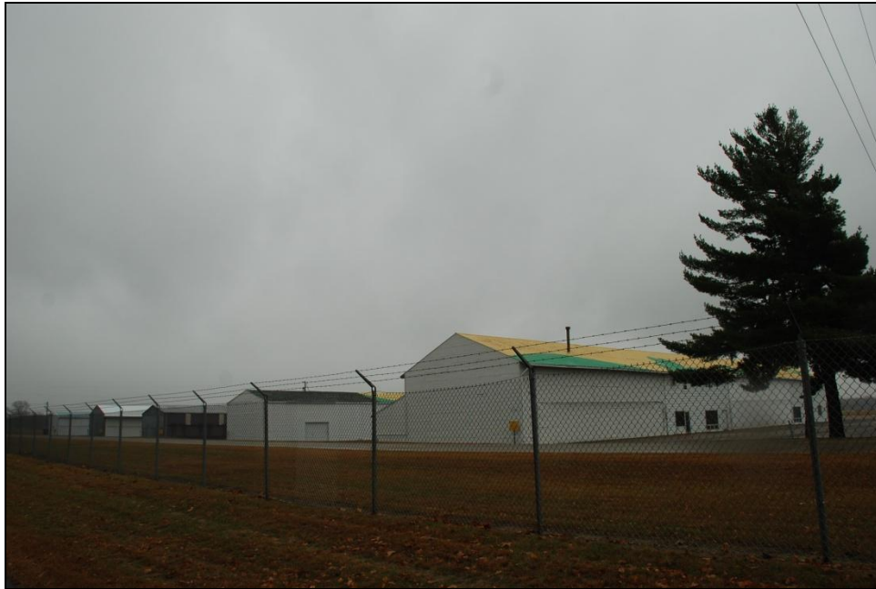
FIGURE 17. HANGARS IN THE DOUGLAS DRIVE AREA OF THE CRYSTAL AIRPORT (HE-CRC-112), FACING NORTHEAST
