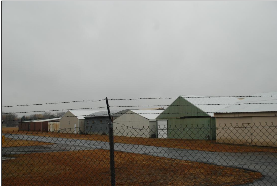
FIGURE 13. HANGARS ON CRYSTAL AIRPORT ROAD AT THE CRYSTAL AIRPORT (HE-CRC-112), FACING NORTHEAST
