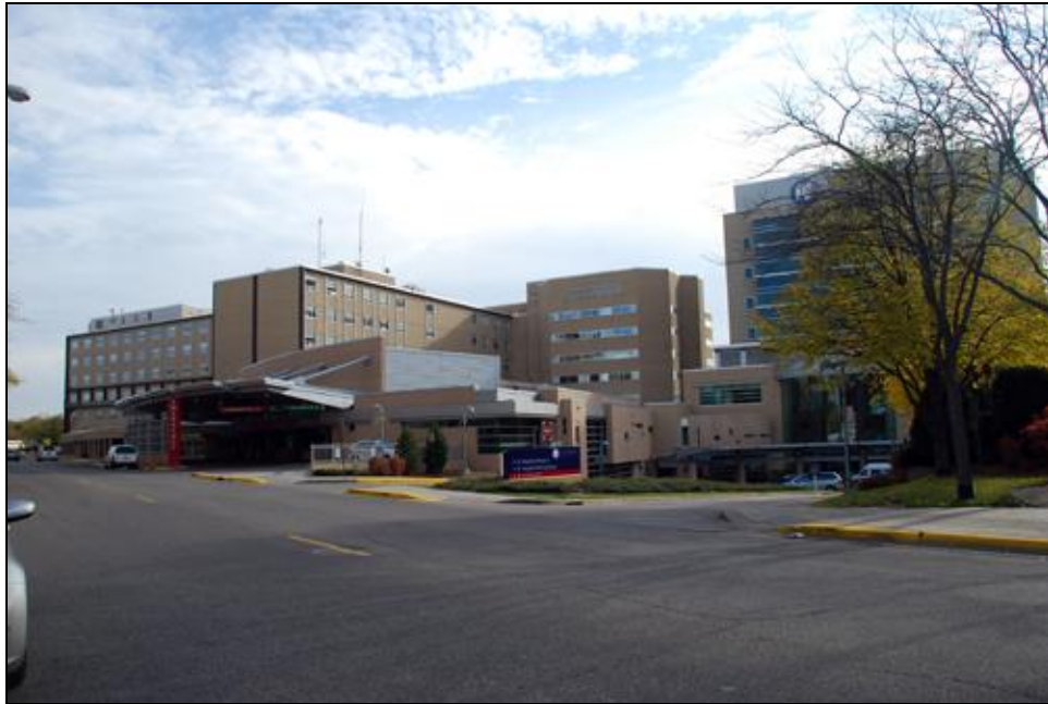
FIGURE 123. VICTORY MEMORIAL HOSPITAL / NORTH MEMORIAL HOSPITAL COMPLEX (HE-RBC-1279), FACING SOUTHEAST
