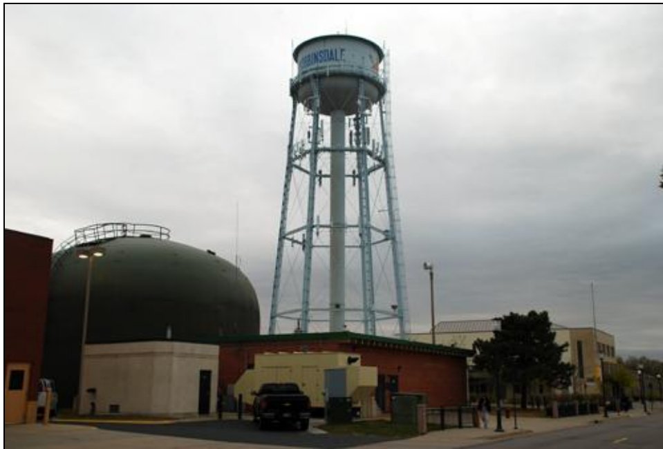
FIGURE 116. VILLAGE OF ROBBINSDALE WATER WORKS (HE-RBC-286), FACING NORTHWEST
