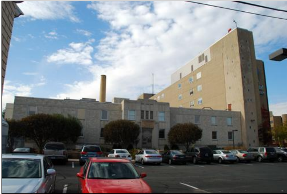
FIGURE 119. VICTORY MEMORIAL HOSPITAL / NORTH MEMORIAL HOSPITAL COMPLEX (HE-RBC-1279), FACING WEST
