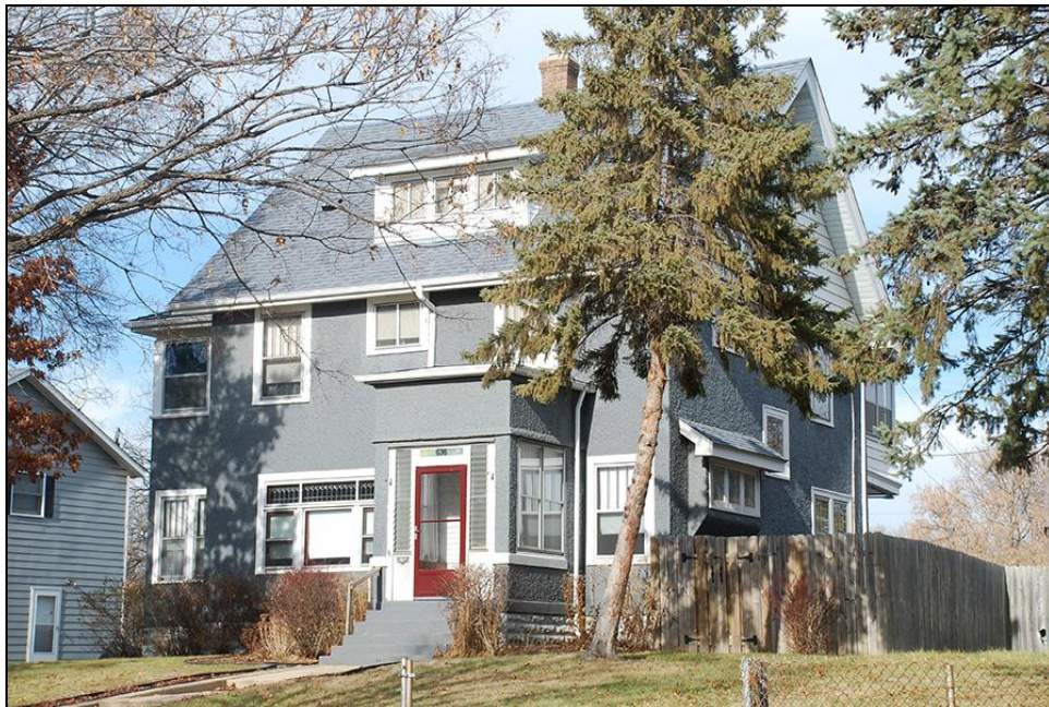
FIGURE 79. EDWARD RAPPAPORT HOUSE (HE-MPC-1600), FACING NORTHWEST
