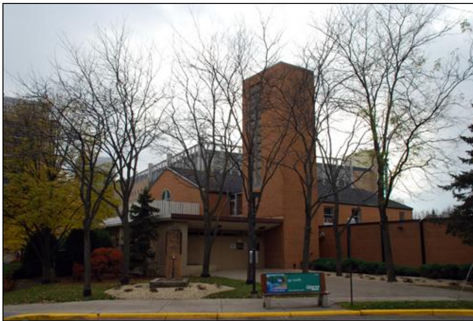
FIGURE 124. VICTORY MEMORIAL HOSPITAL / NORTH MEMORIAL HOSPITAL COMPLEX (OLIVET BAPTIST CHURCH) (HE-RBC-1279), FACING SOUTHWEST
