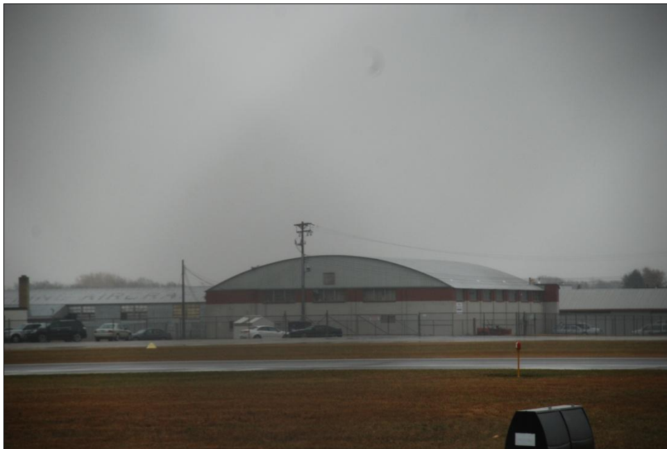
FIGURE 14. HANGARS ON CRYSTAL AIRPORT ROAD AT THE CRYSTAL AIRPORT (HE-CRC-112), FACING SOUTHEAST
