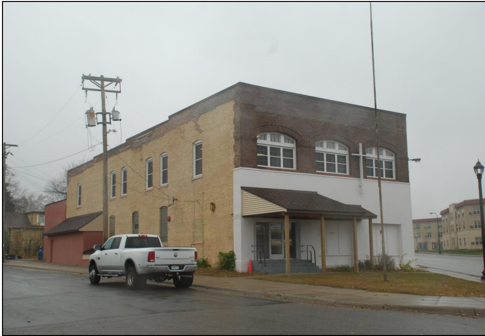
FIGURE 110. STATION 25 MINNEAPOLIS FIRE DEPARTMENT / AMERICAN LEGION NORTH SIDE POST NO. 230 (HE-MPC-8034), FACING NORTHWEST
