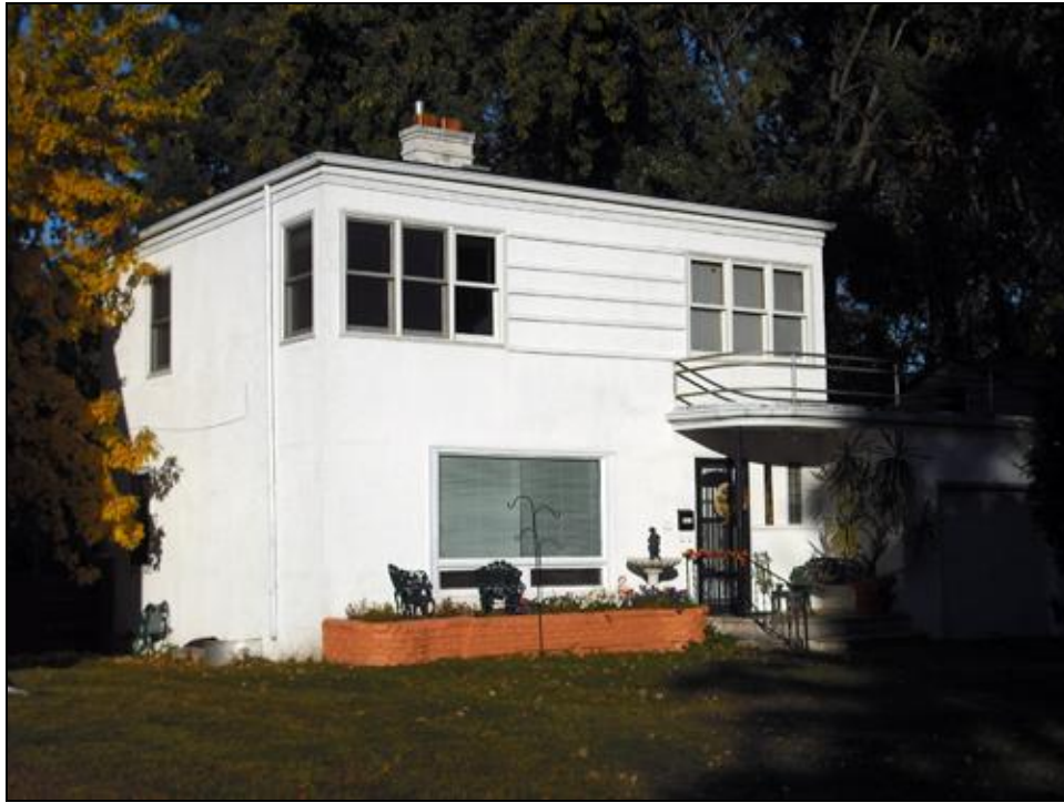
FIGURE 50. BENHARDT BUHRT HOUSE (HE-GVC-350), FACING NORTHWEST
