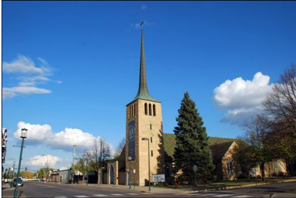
FIGURE 132. SACRED HEART CATHOLIC CHURCH (HE-RBC-1462), FACING NORTHEAST
