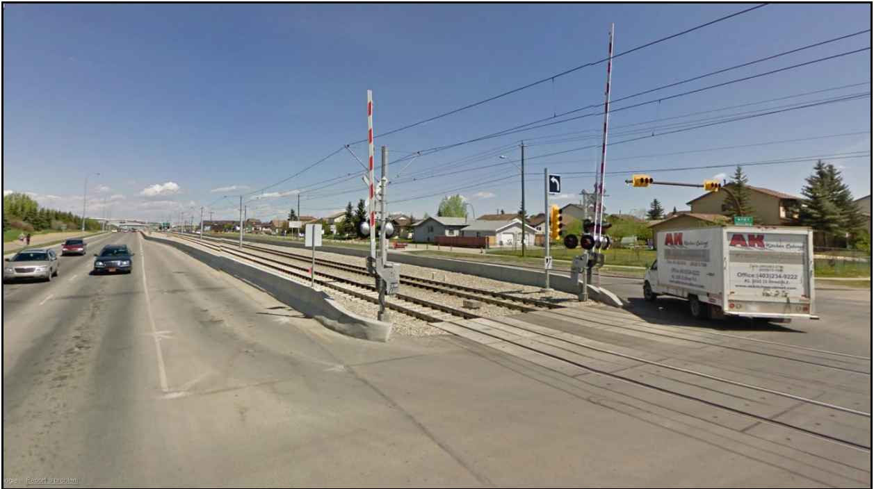
Figure 3. Center-Running Gated LRT Guideway 36 th Street NE/39 th Avenue NE intersection. Source: Google Streetview
