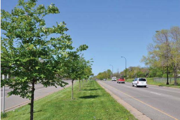
Figure 28 - View of planted median along TH 55 looking west
