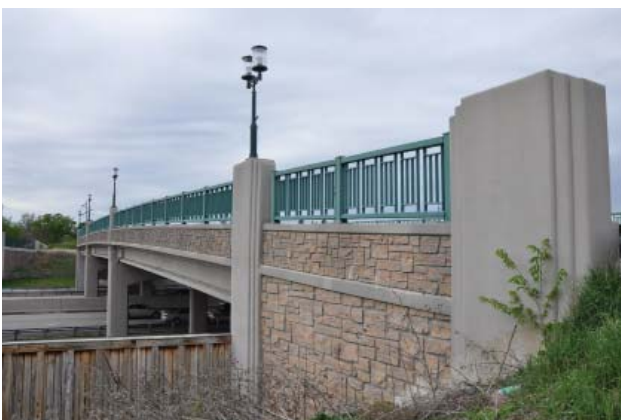
Figure 9 - View of West Broadway Avenue bridge over TH 100
