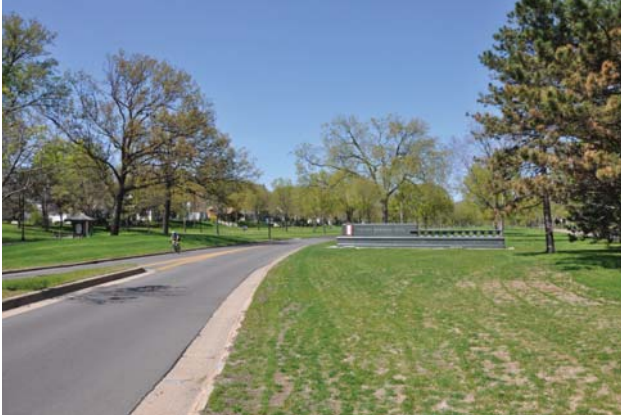
Figure 18 - View Victory Memorial Drive looking north
