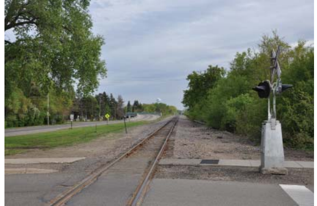
Figure 20 -View south along BNSF right of way from 45 1/2 Avenue. West Broadway Avenue at left.
