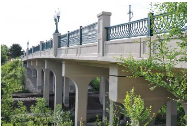
Figure 16 - View of Plymouth Avenue Bridge over Bassett Creek and BNSF railroad
