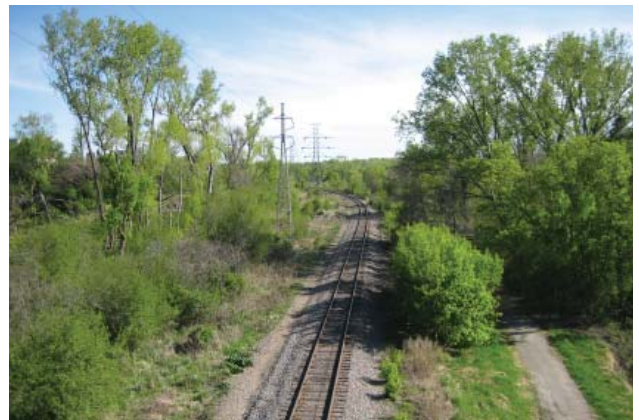
Figure 30 - View of BNSF right of way looking south from the Plymouth Avenue Bridge. Theodore Wirth Park and golf course is on the right.
