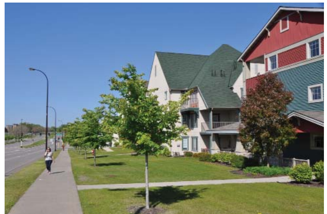
Figure 53 - View west along the north side of TH 55 east of Bryant Avenue.
