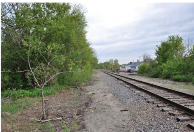
Figure 17 - View south along BNSF right of way south of Corvallis Avenue.
