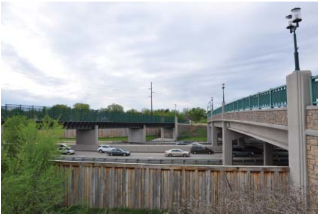
Figure 21 - View north across TH 100. BNSF bridge at left. West Broadway Avenue bridge at right.
