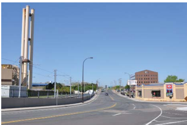
Figure 54 - View west along 6th Avenue from the 5th St intersection. HERC and future Interchange site at left.
