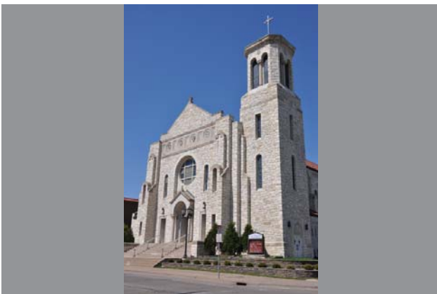
Figure 22 - View of Church of St. Anne
