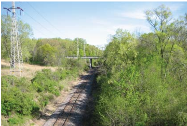
Figure 29 - View of BNSF right of way looking south from the Golden Valley Road Bridge. Theodore With Parkway Bridge is in the distance.
