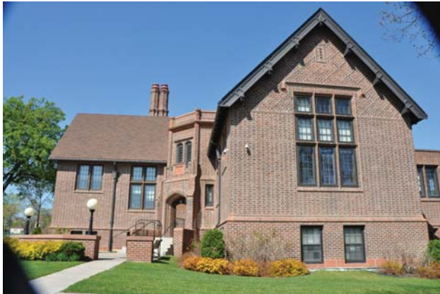
Figure 32 - View of Sumner Library at the northwest corner of TH 55 and Van White Memorial Boulevard
