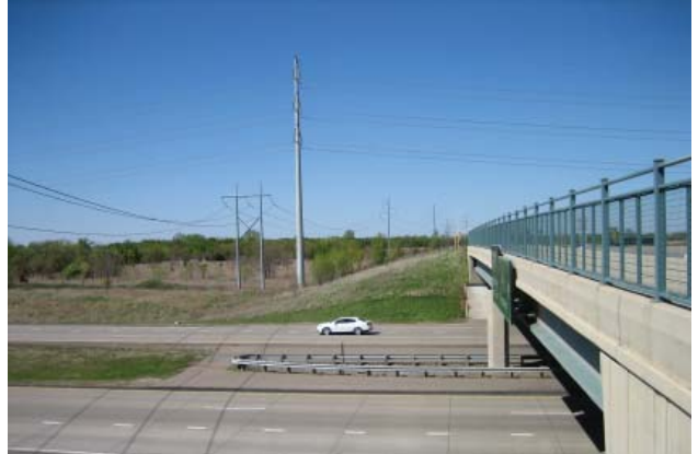
Figure 4 - View of West Broadway Bridge over TH 610
