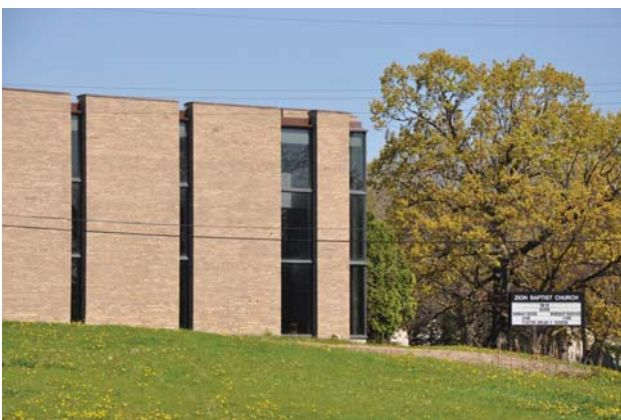
Figure 32 - View of Zion Baptist Church from TH 55
