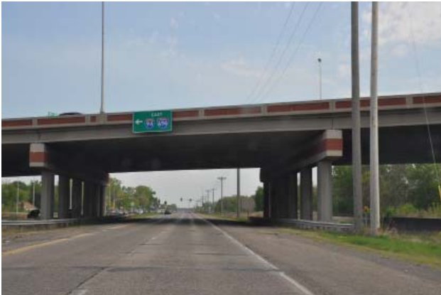
Figure 5 - View of Interstate 94 bridge over BNSF railroad and Bottineau Boulevard from Bottineau Boulevard looking south
