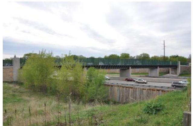
Figure 8 - View of BNSF railroad bridge over TH 100
