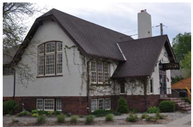
Figure 10 - View of Historic Robbinsdale Public Library
