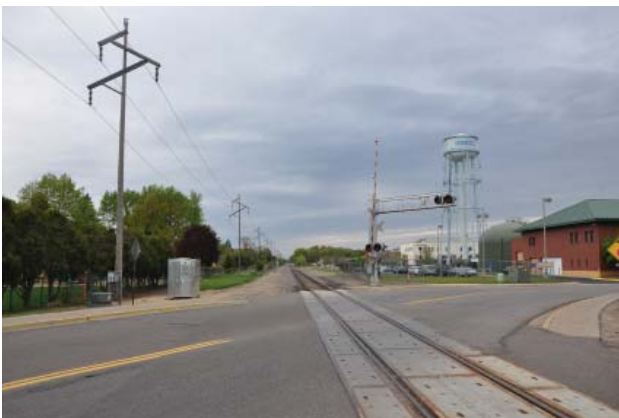
Figure 23 - View north along BNSF right of way from Noble Avenue.
