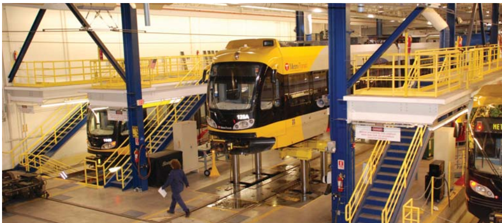
Interior of Franklin OMF (maintenance area).
