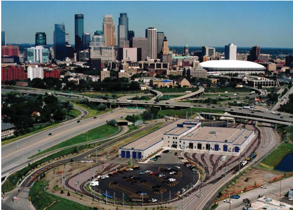
Franklin OMF serving the Blue Line (Hiawatha LRT).
