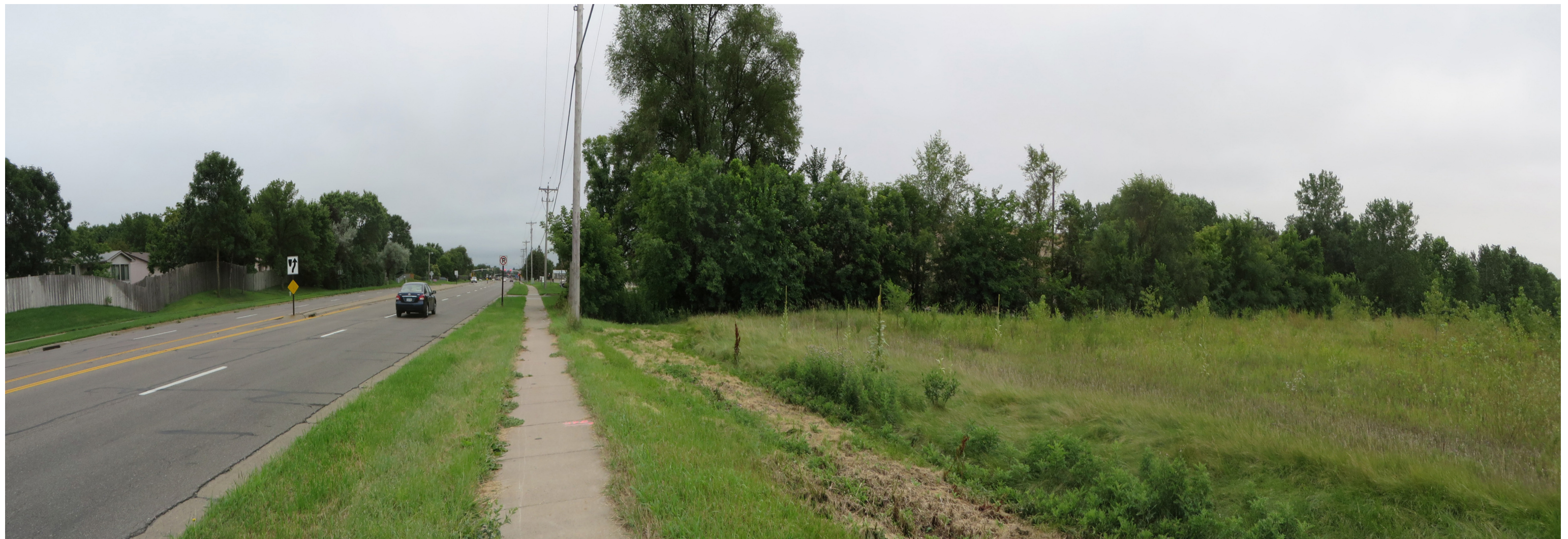
View looking south from West Broadway Ave toward proposed TPSS BL412 site
