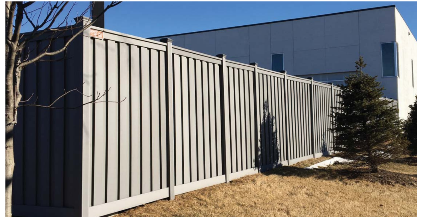
Public Works building in Crystal
