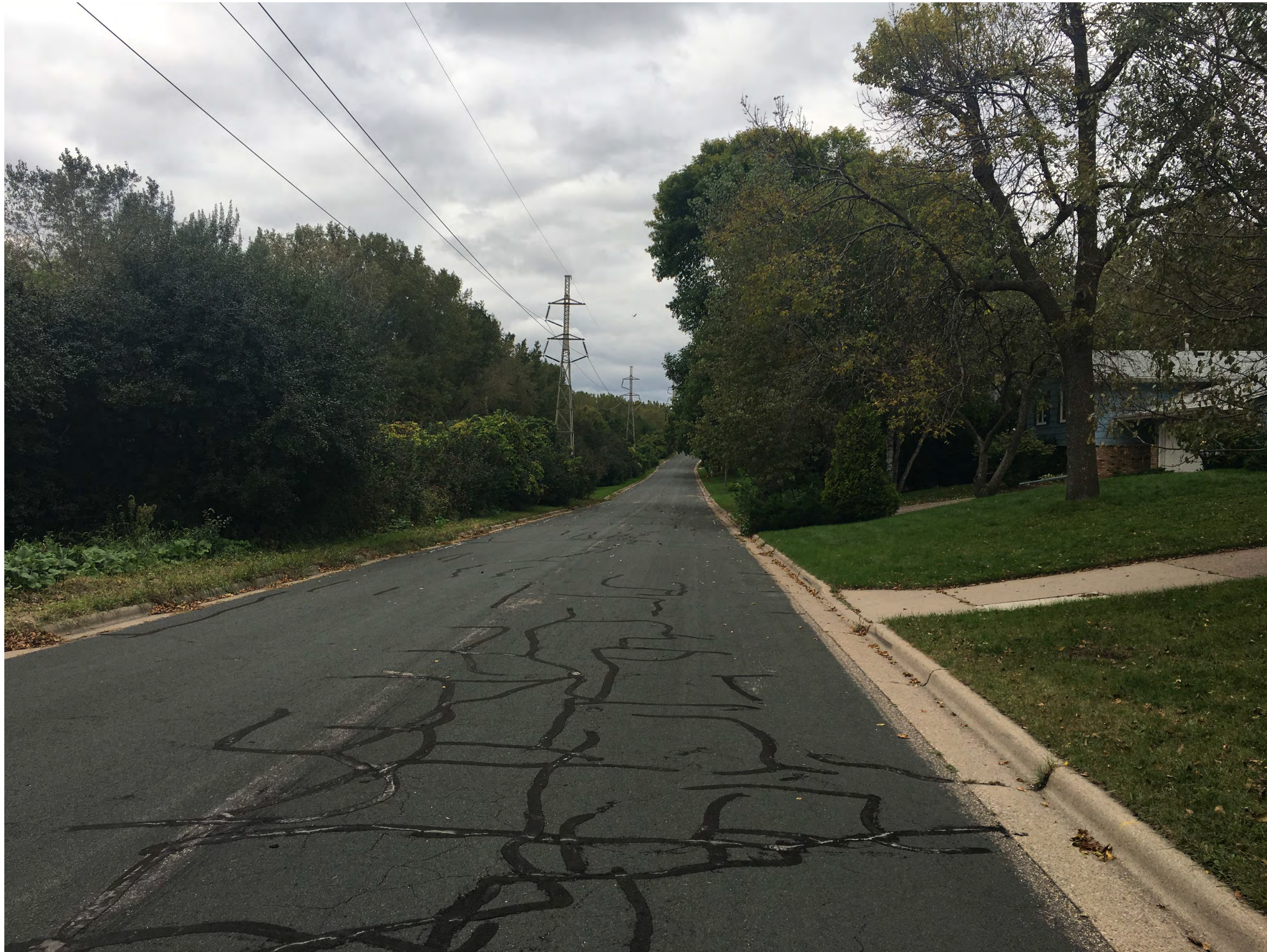
View along Kewanee Way Looking North (at South End)
