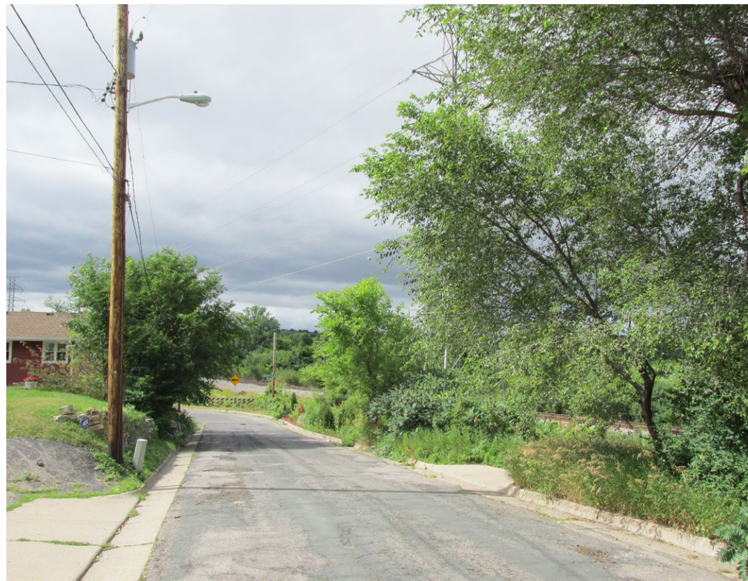
View looking south down Xerxes Ave N
