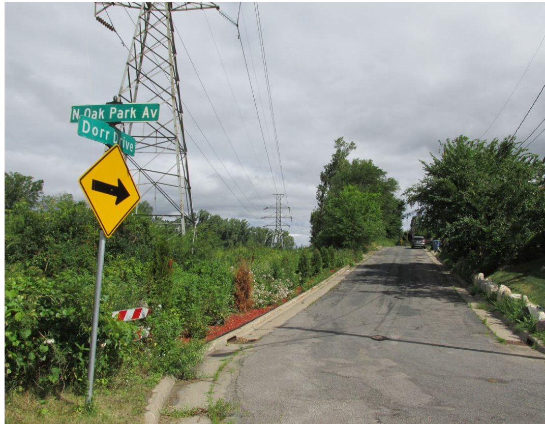
View looking north down Xerxes Ave N toward proposed TPSS BL403 site
