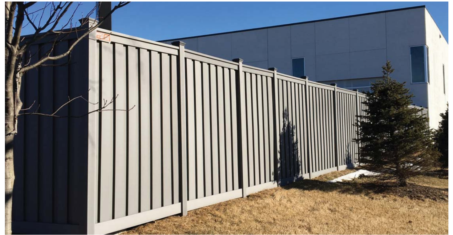
Public Works building in Crystal
