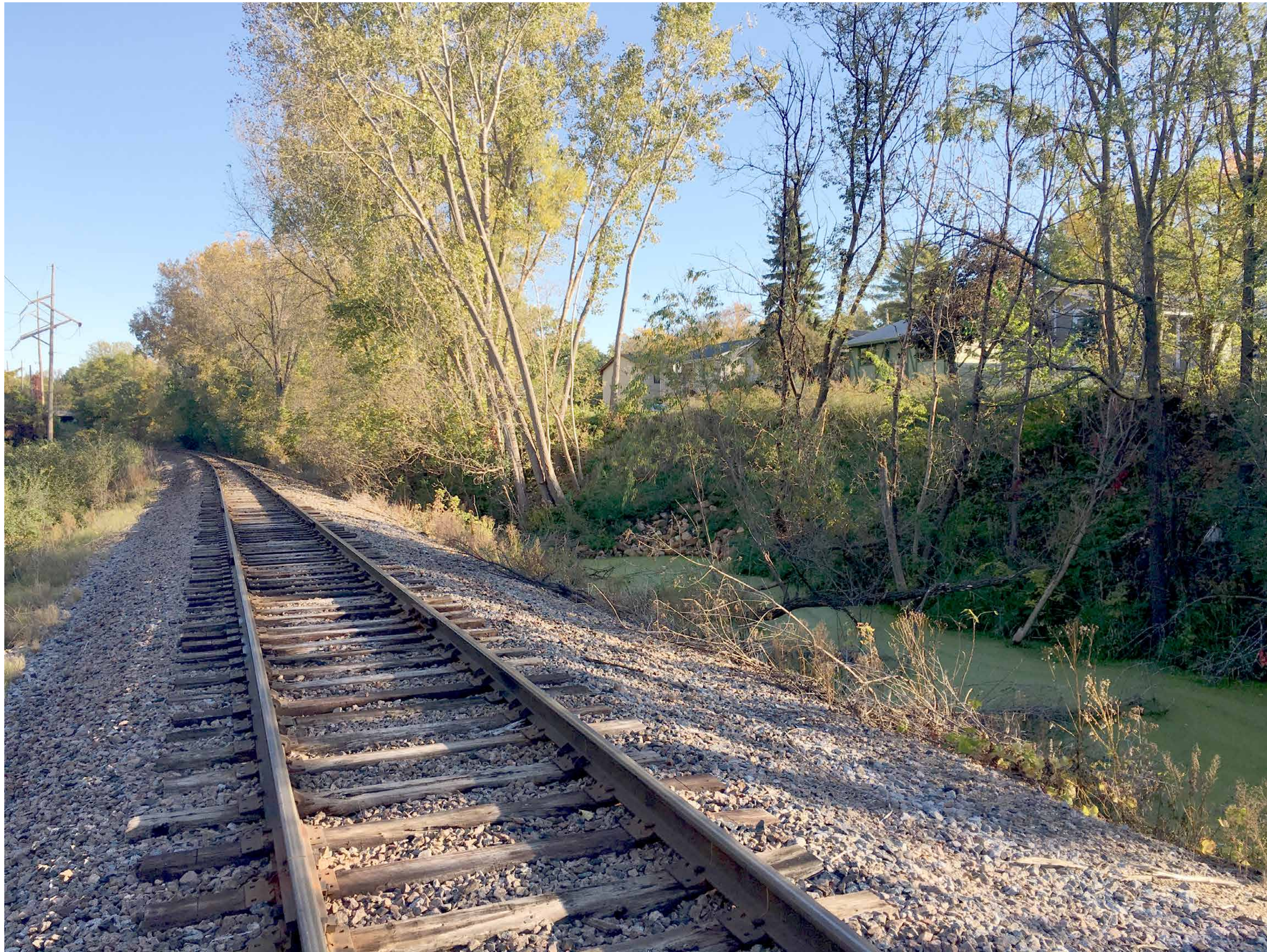
View from West Side of Rail Corridor Looking North
