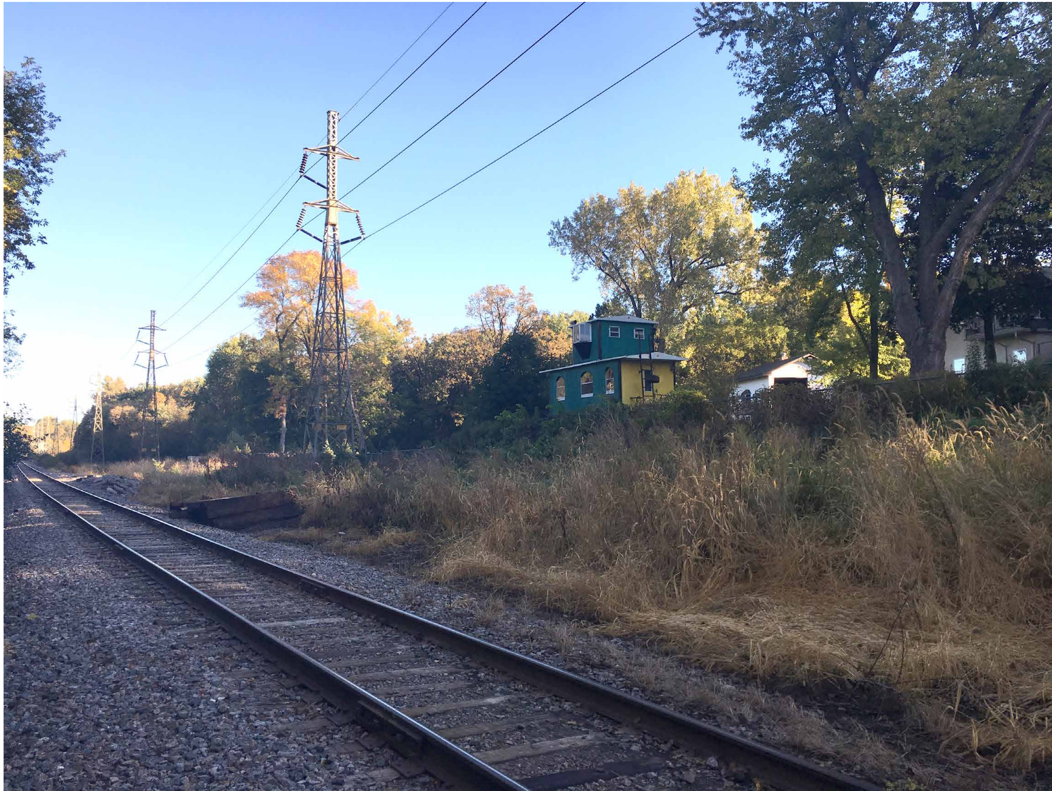
View from the West Side of the Rail Corridor Looking North
