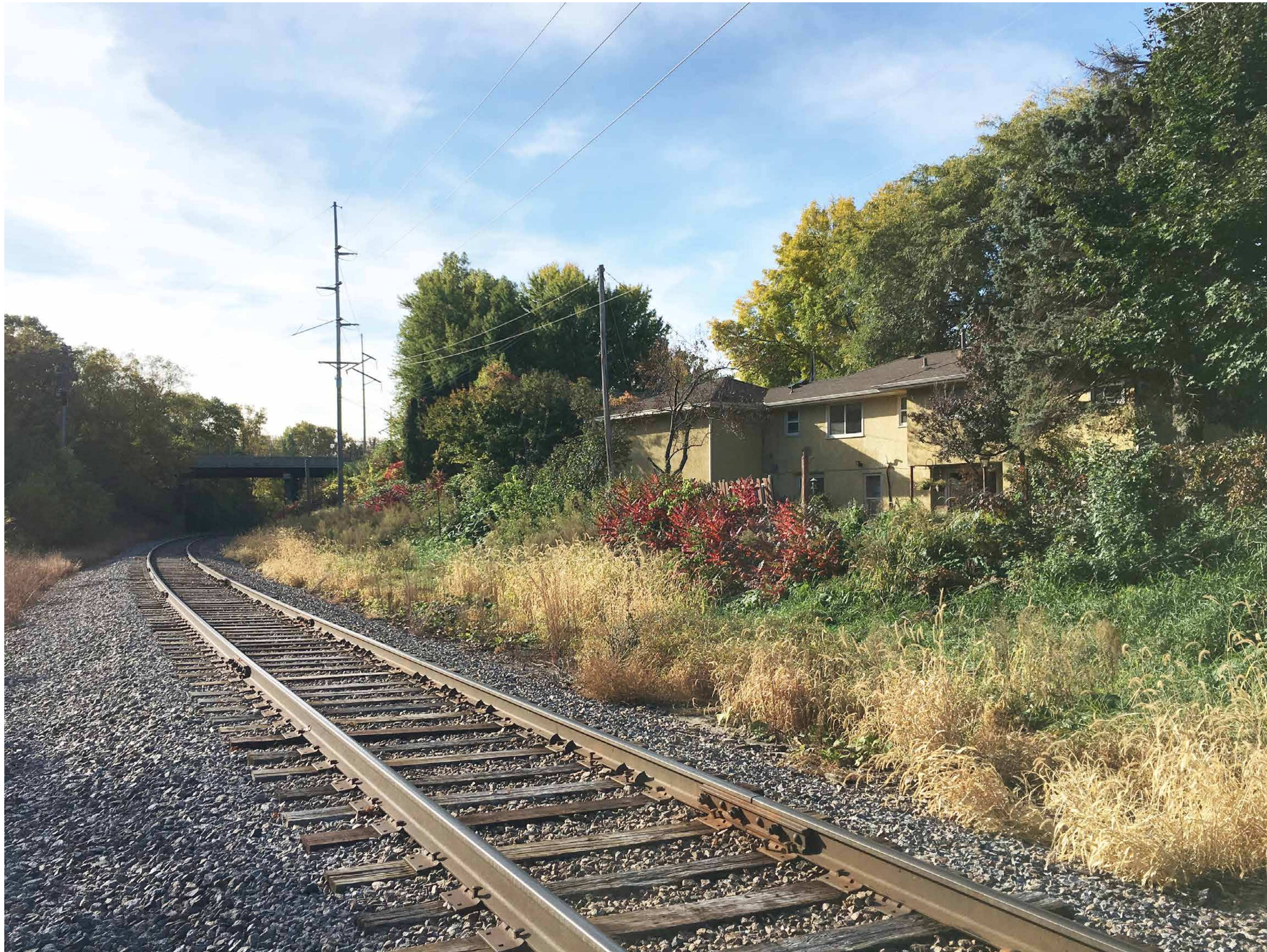
View from East Side of Rail Corridor Looking South
