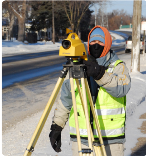
Jeremy Honga of Sambatek does survey work on the Blue Line Extension LRT Project along Broadway Avenue in Robbinsdale
