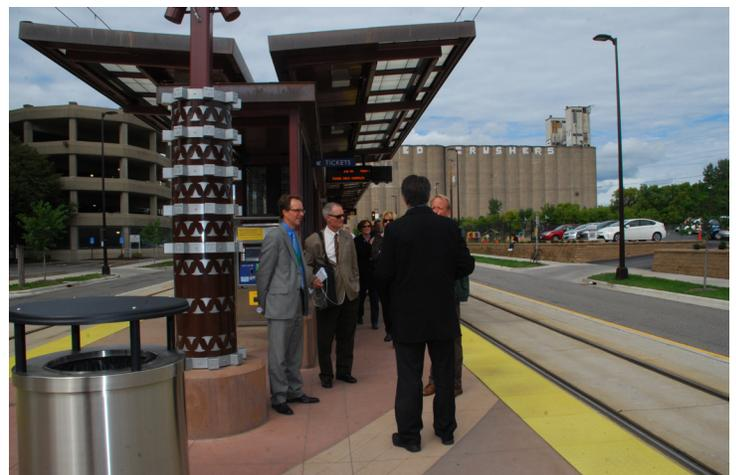
*Prospect Park Station on the METRO Green Line (top) is an example of the center-platform design. A single platform (above) serves trains traveling in both directions.*
