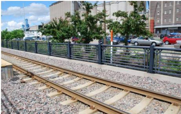
Safety railings near stations prevent pedestrians from walking onto the light rail tracks.
