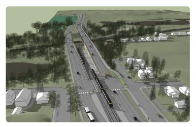
Looking west toward Golden Valley, Blue Line Extension LRT trains would operate in the middle of Highway 55 until reaching BNSF Railway right-of-way where the LRT trains would descend to operate on the east side of the freight tracks for eight miles.
